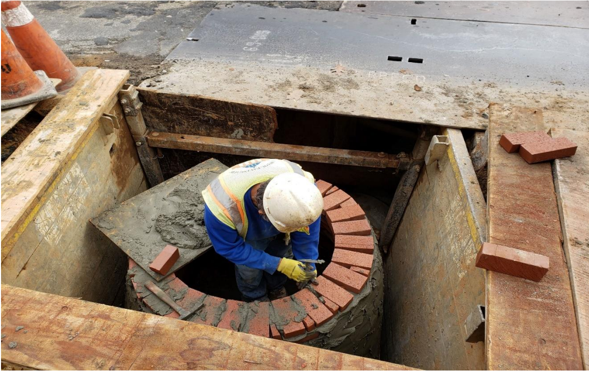
12/31/2019- Building Manhole C-2 near the NW corner of 3 rd and M St. NW. (East view)
