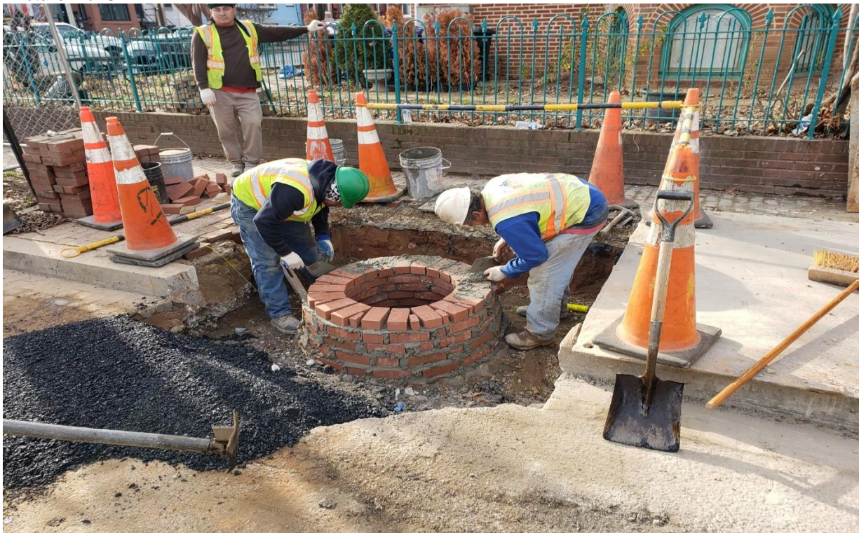
01/02/2020- Building up Manhole C-2, near 3 rd and M St. NW.
