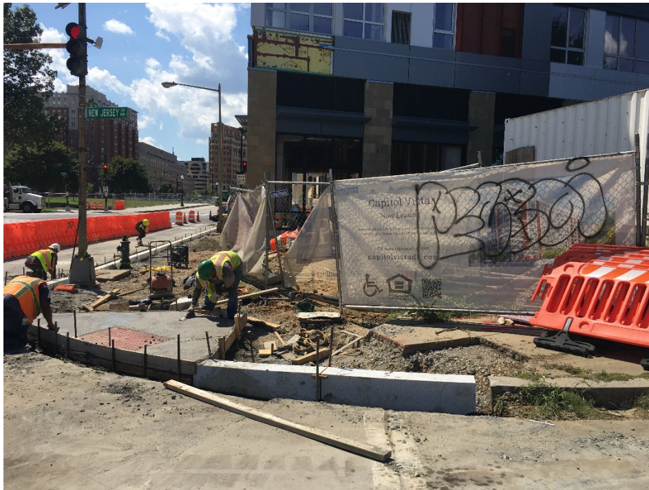
Picture No. 3 - 08/18/2020 – Installation of wheelchair ramp at the intersection of NJ Ave and H St. (West View)
