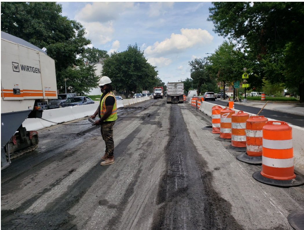
08/20/2020 – Pavement milling in progress along NY Ave between 1 st St. and NJ Ave St. (East View)
