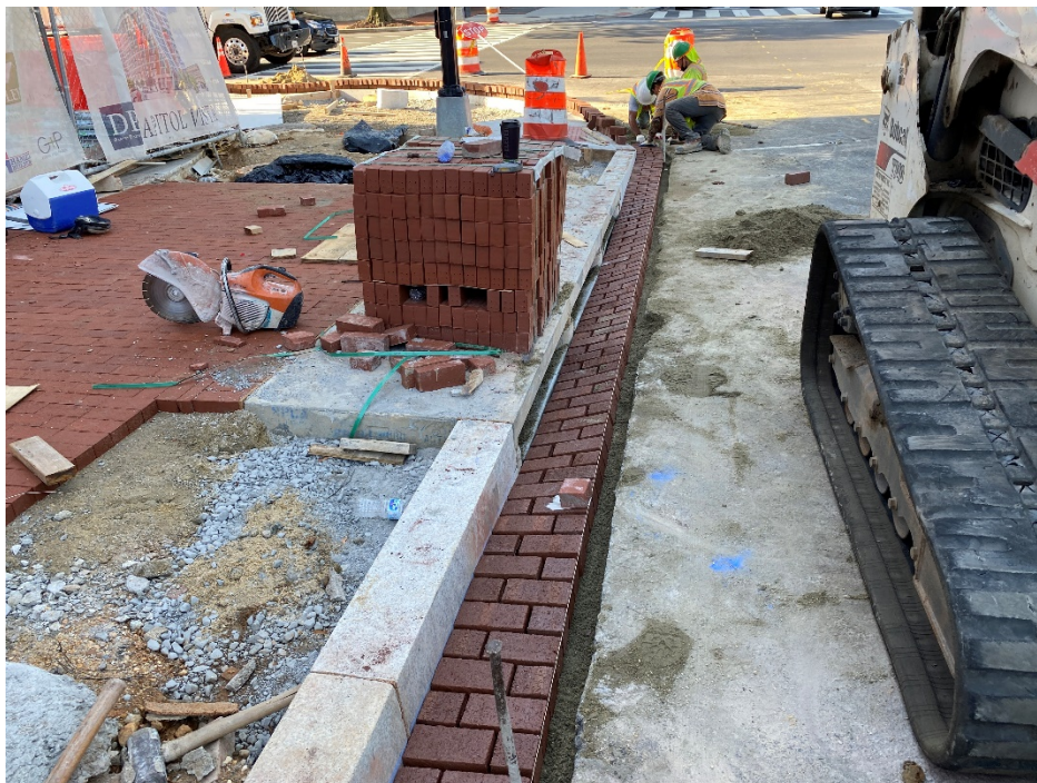
Picture No. 6 – 08/20/2020 – Installation of brick gutter in progress along 2 nd St. and H St. (South View)
