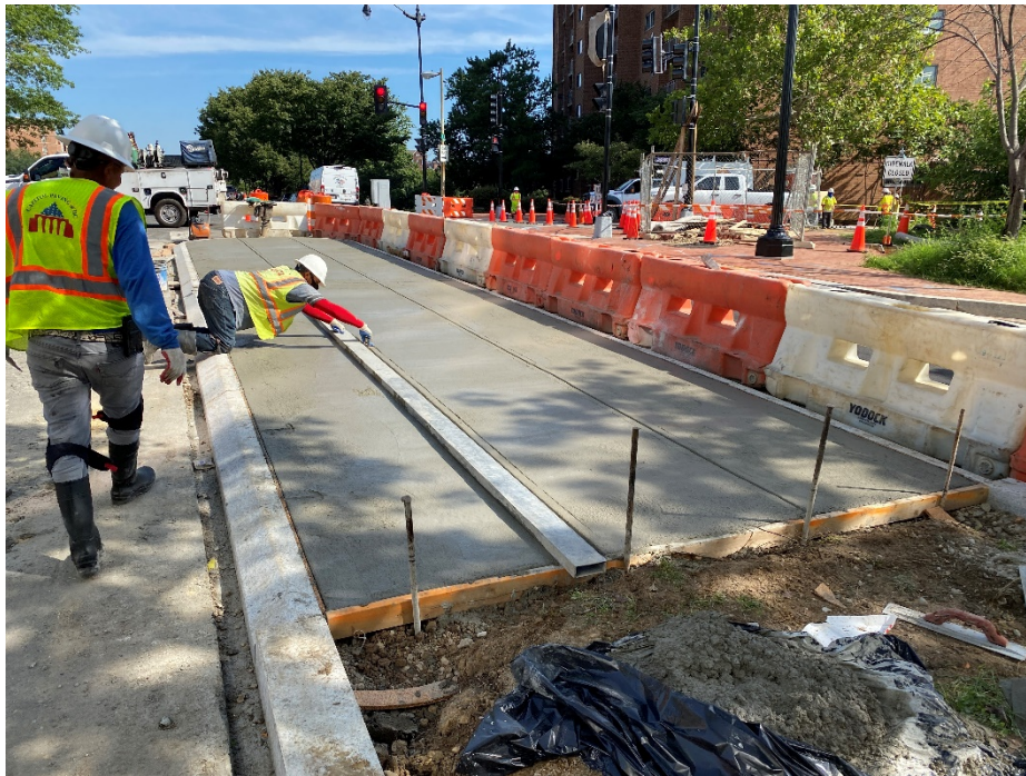
Picture No. 7 – 08/20/2020 – PCC base for the median along NJ Ave and I St. (North View)
