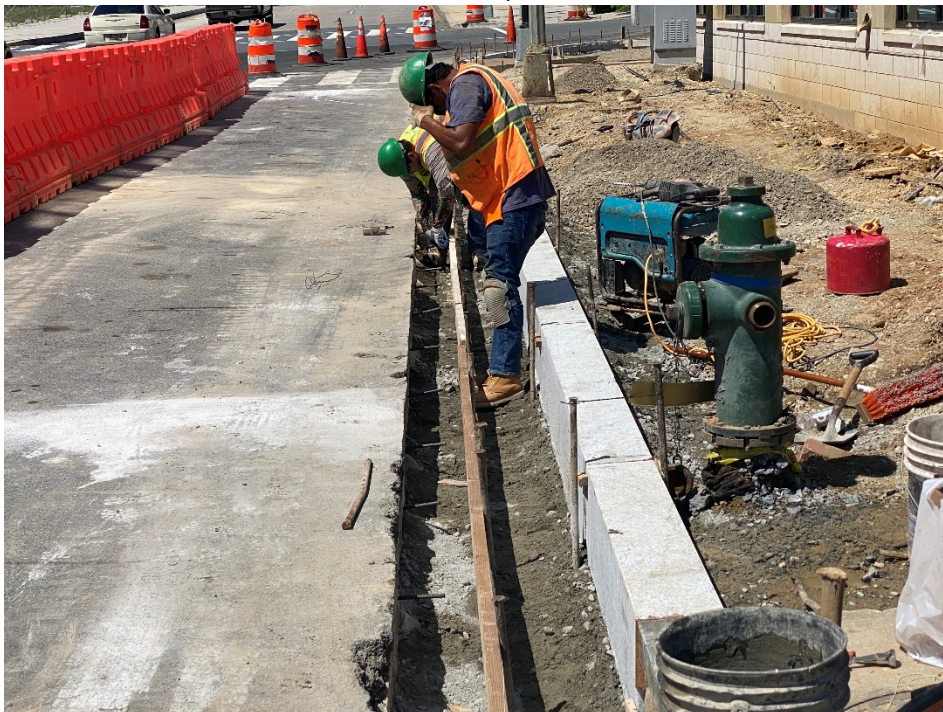
Picture No. 4 – 08/18/2020 – Installation of brick gutter in progress along H St. between NJ Ave and 2 nd St. (West View)
