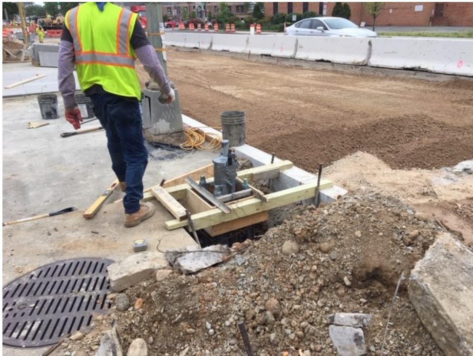
Picture No. 11 – 05/21/2020 – Traffic signal foundation installation at Sta. 319+10 (East View)
