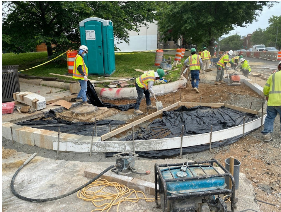
Picture No. 9 – 05/21/2020 – Wheelchair ramp formed at NE corner of NY Ave. and Kirby (East View)
