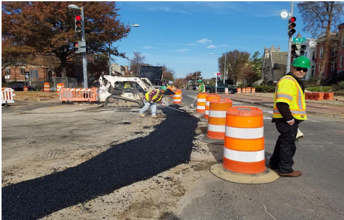
11/15/2019- Repairs to the roadway/trench line excavated for conduit installation at NJ Ave between NY & M Morgan St. NW. (North View)
