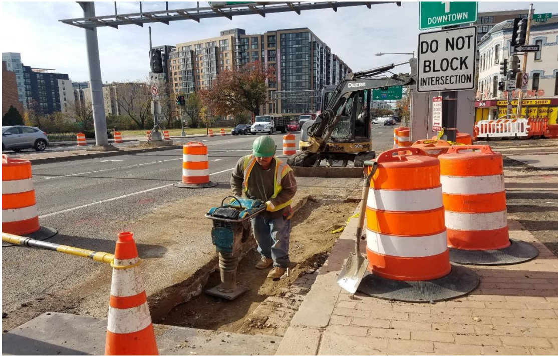
11/15/2019- Compaction to the soil backfill for TL/SL condits at NJ & NJ Ave. NW ( West View)
