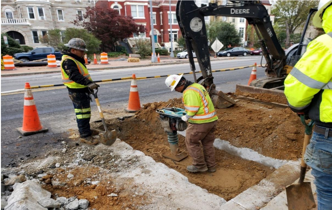
11/12/2019- Compaction to the soil backfill for water service line installed at 1252 NJ Ave. NW. (SE view)
