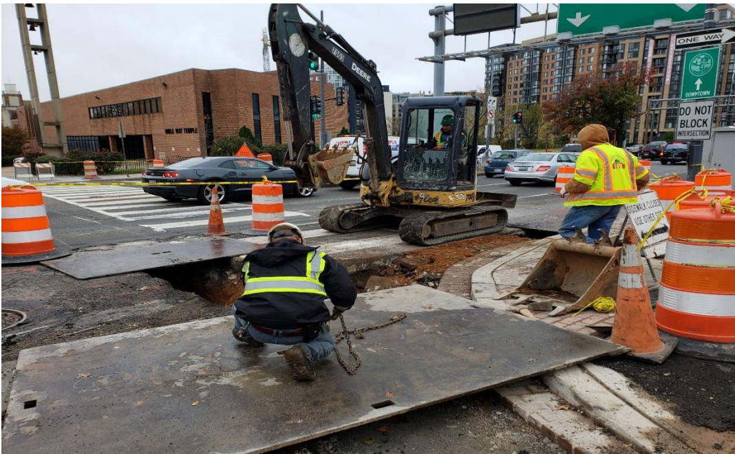
11/12/2019-Safety measures to the trench excavated for electrical conduits at NW corner of NJ & NY. (SW view)
