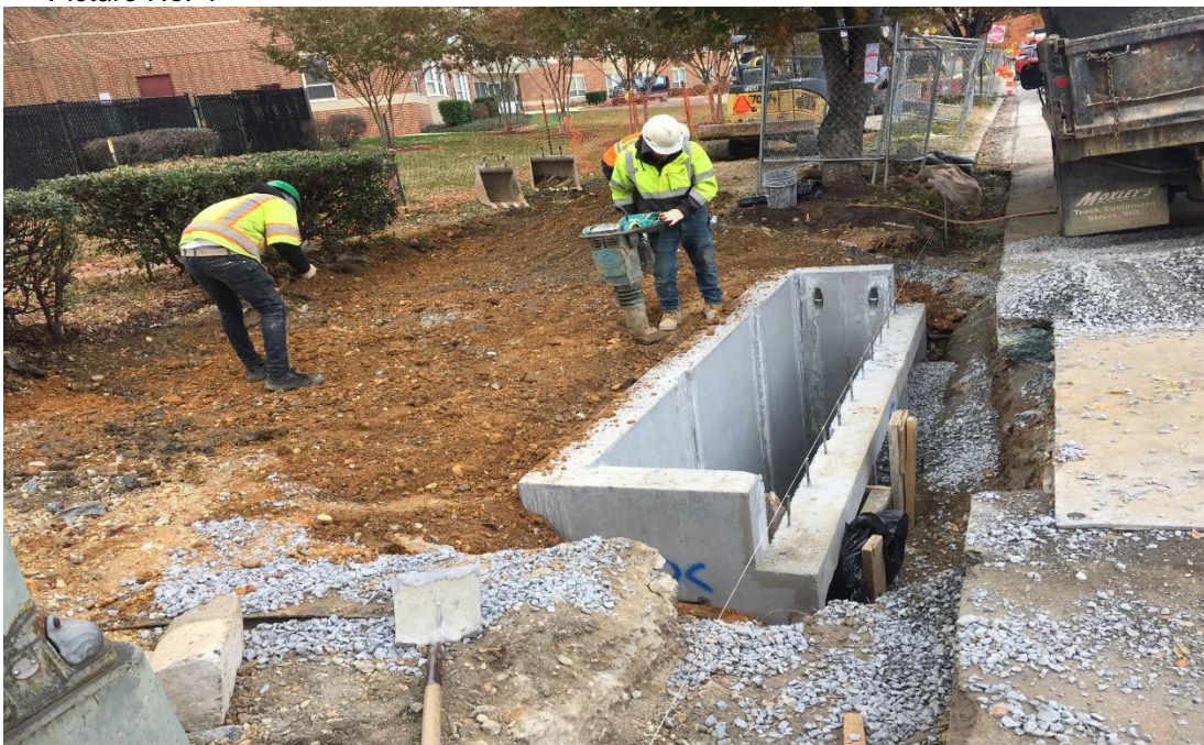
11/14/2019- Installing catch basin R1 along on west side NJ Ave between K St and L St (north View)
