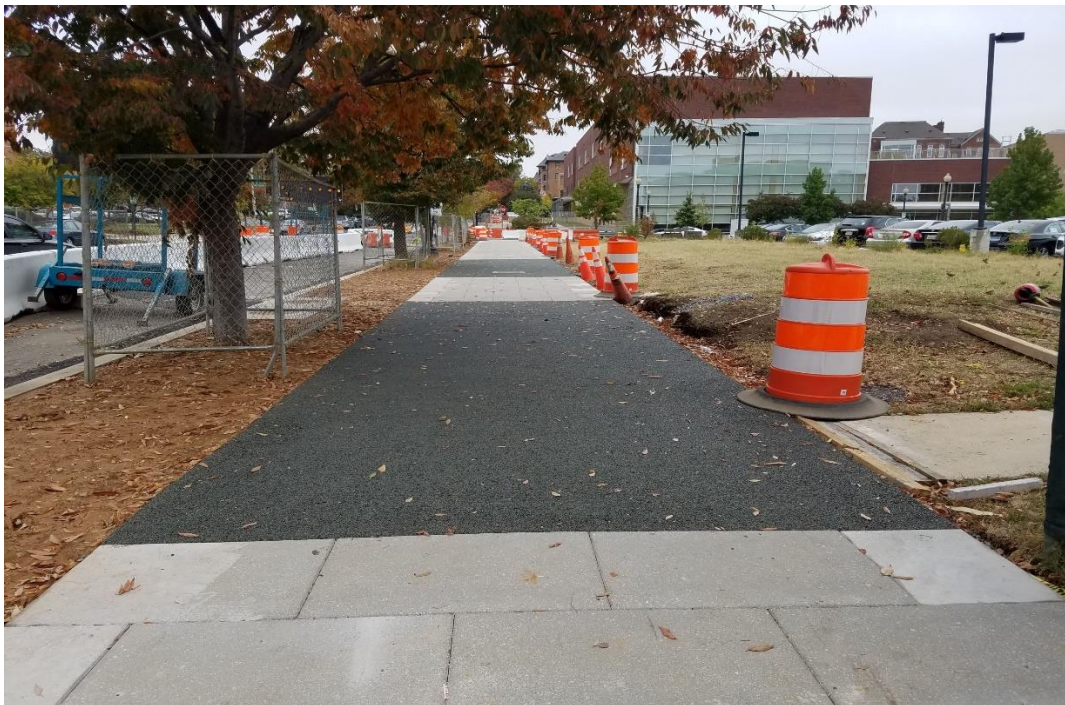
10/22/2019- Newly constructed flexipave at East side of NJ Ave. NW between L & K St. NW. (North view)
