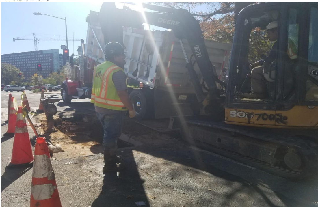
10/24/2019- Excavation work to install tie-in from new-to-new water main at 3 rd & M St. NW. (SW view)
