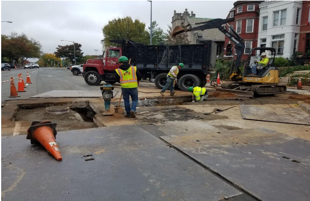
10/22/2019- Soil backfill for connect pipe between MH F4 & CB F2 at New Jersey Ave. NW. (North view)
