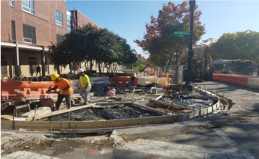
10/21/2019- Formwork prep. For WCR at SE corner of New Jersey & Pierce St. NW (South View)
