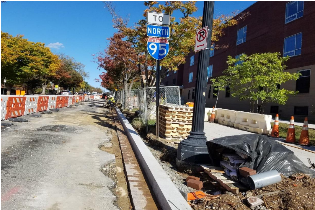
10/23/2019-Newly constructed granite curb & brick gutter at East side of NJ Ave. b/n L & Pierce St.
