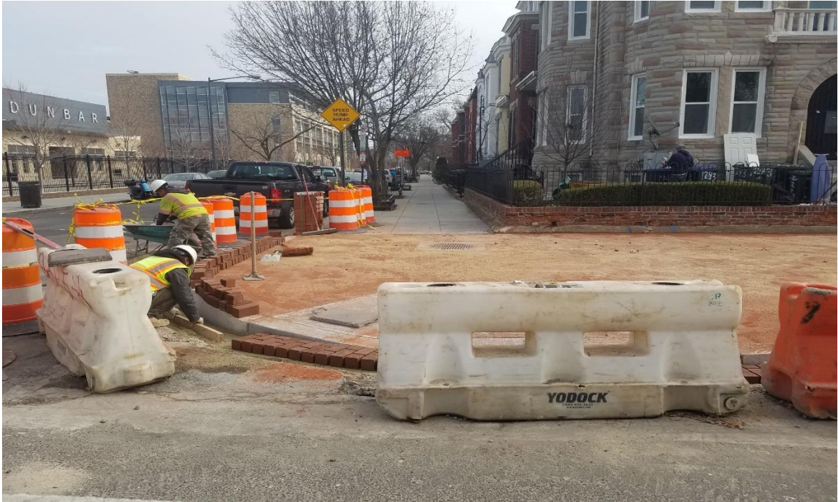
01/24/2020- Brick gutter construction at 3 rd & N St. NW. (East View)
