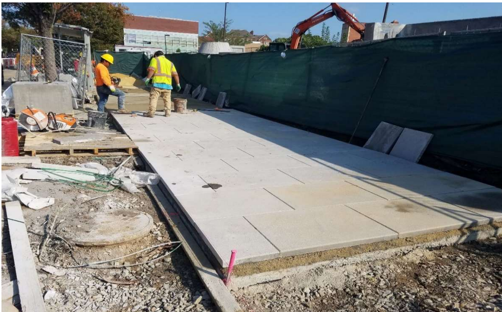
10/01/2019-Block Paver Sidewalk Construction at East side of NJ Ave. NW b/n K & L St. (North View)
