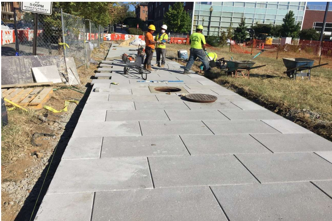
10/04/2019 – Installation of block sidewalk on PCC base on NJ Ave (east side) between K St and L St (north view)
