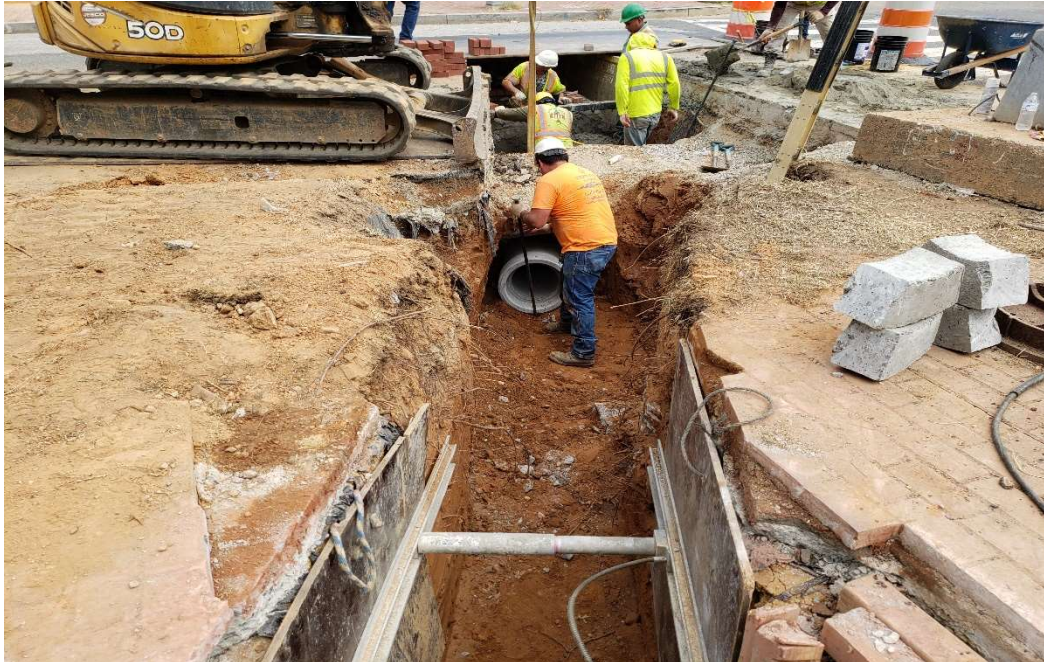
10/02/2019 – Installation of 15 inch PCC connect pipe from CB-E1 to MH-F2 near NJ Ave and M St NW (East View)
