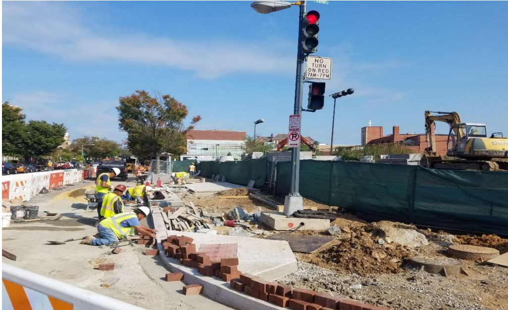
10/01/2019- Brick gutter construction at NE corner of New Jersey Ave. & K St. NW. (North View)
