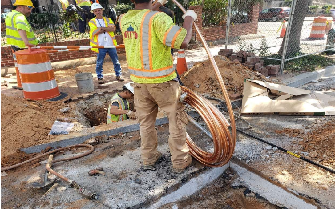
10/04/2019- Replacing water service connections on NJ Ave between Morgan St and N St (east view)
