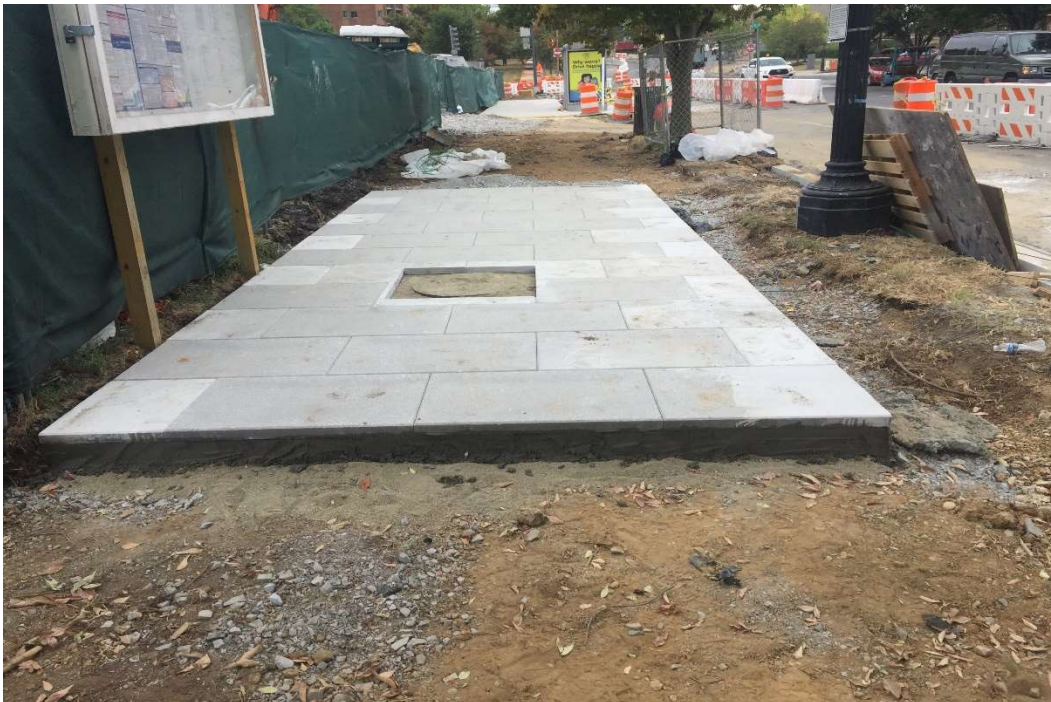
10/03/2019 – Block sidewalk on PCC base along NJ Ave (east side) between K St and L St. (South View)
