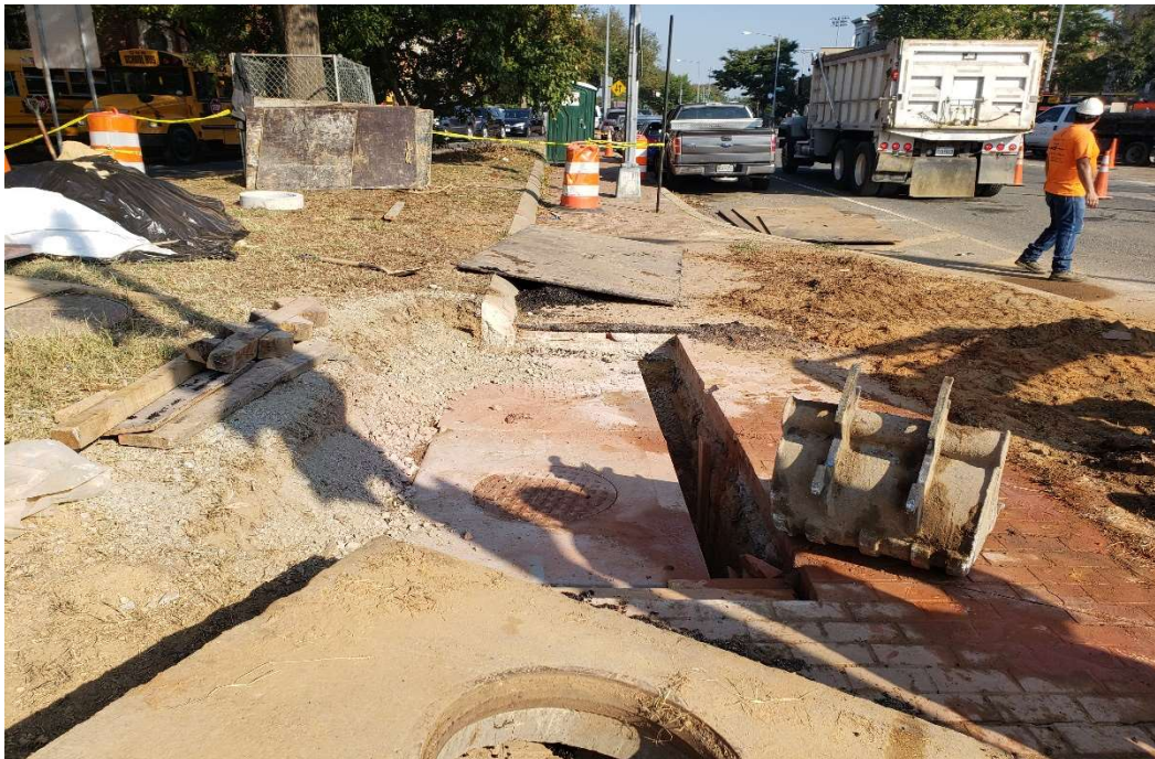
10/02/2019 – Installed catch basin E1 near the northwest corner of NJ Ave and M St (north view)
