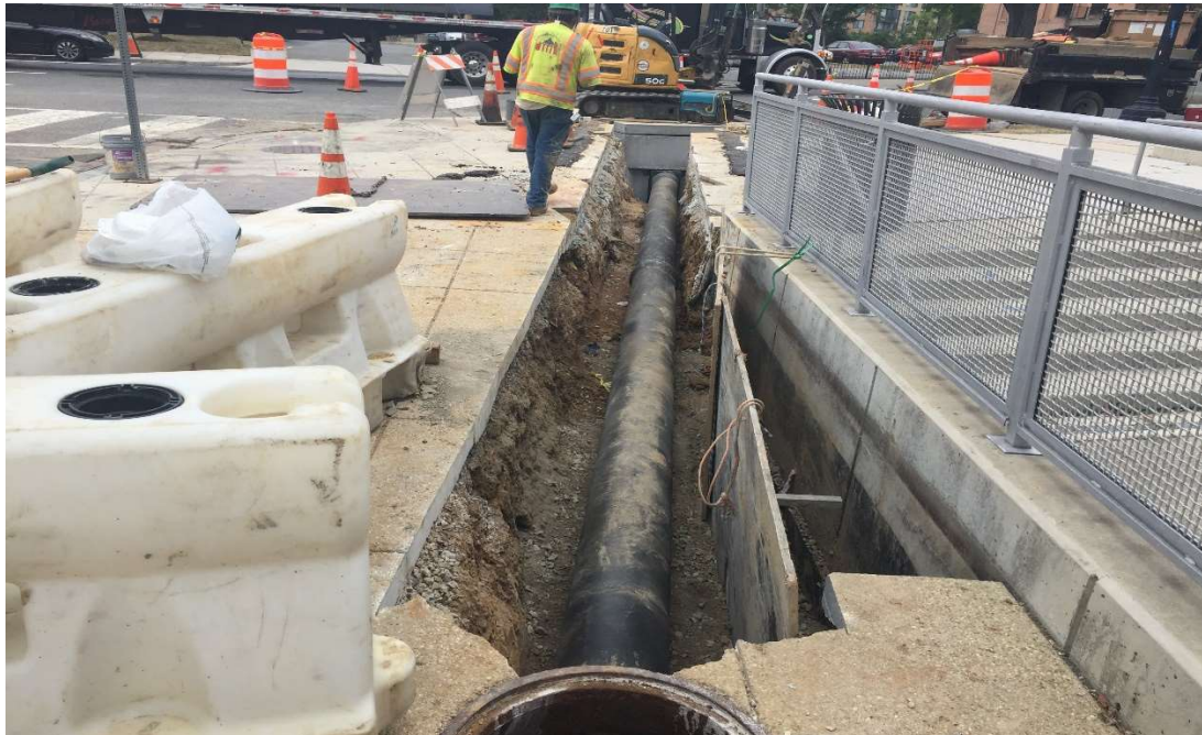
10/03/2019- Installation of 12-inch ductile iron pipe from CB-P to existing manhole (west view)
