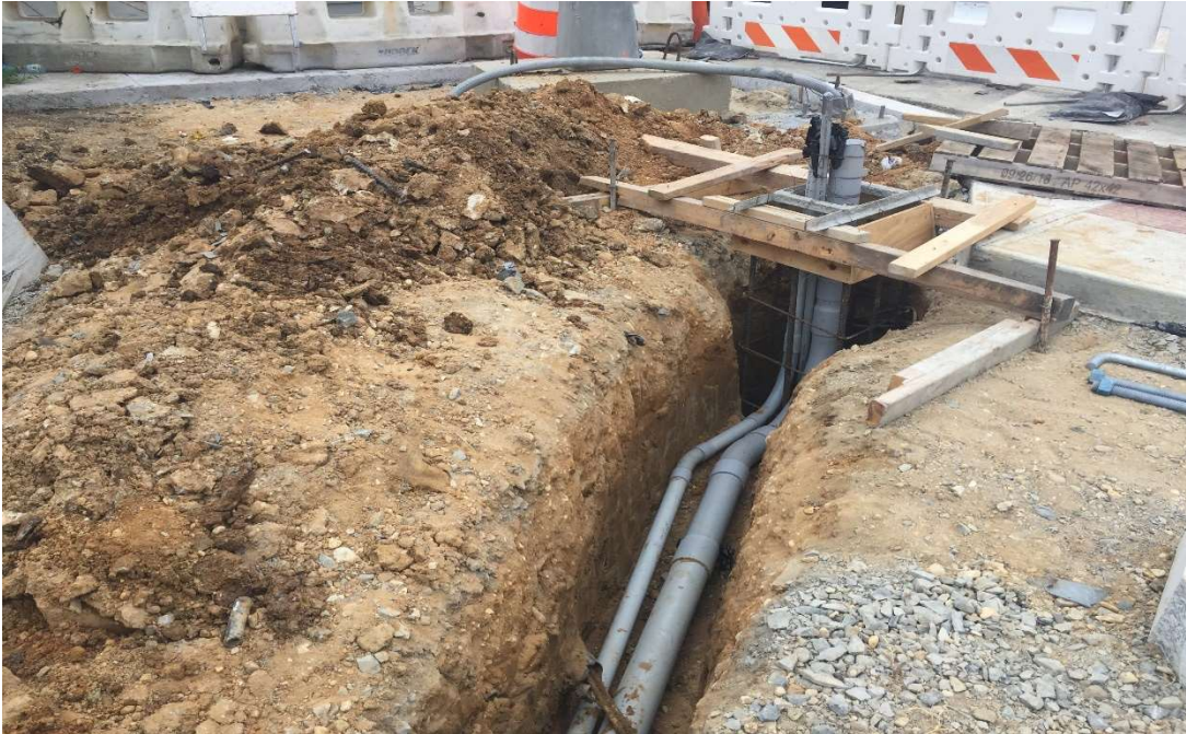
10/03/2019- PVC electrical conduits for traffic signal foundation at the corner of NJ Ave and K St (southeast view)
