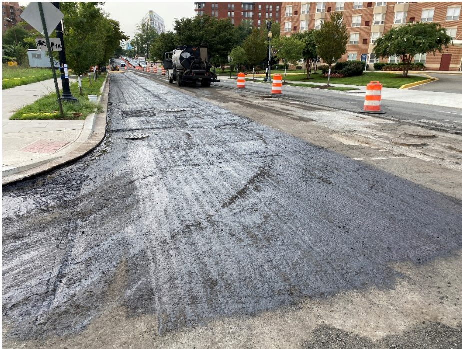
Picture No. 9 – 09/16/2020 – Placement of tack coat along NJ Ave between K St. and NY Ave (South view)
