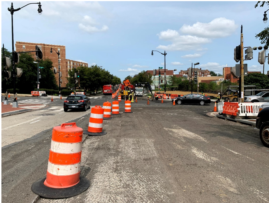
Picture No. 3 - 09/14/2020 – Pavement milling in progress at the intersection of NJ Ave and K St. (North View)
