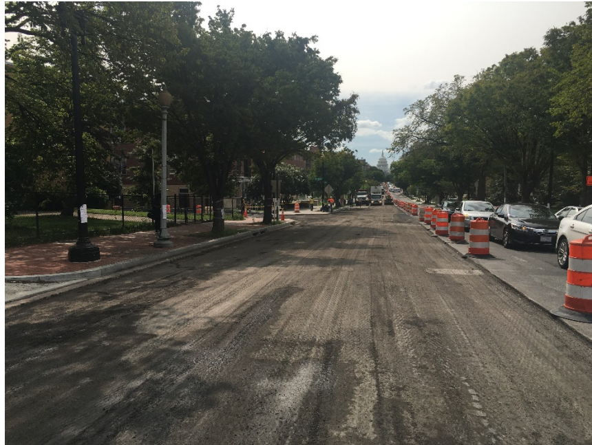
Picture No. 1: 09/14/2020 – Pavement milling along NJ Ave between NY Ave and L St St. (South View)
