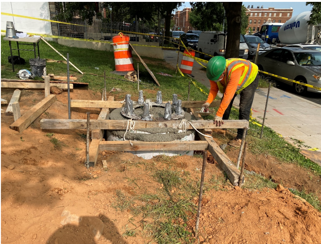
09/15/2020 – Drilled shaft installation in progress at NY Ave and Kirby St. for overhead sign structure (East View)
