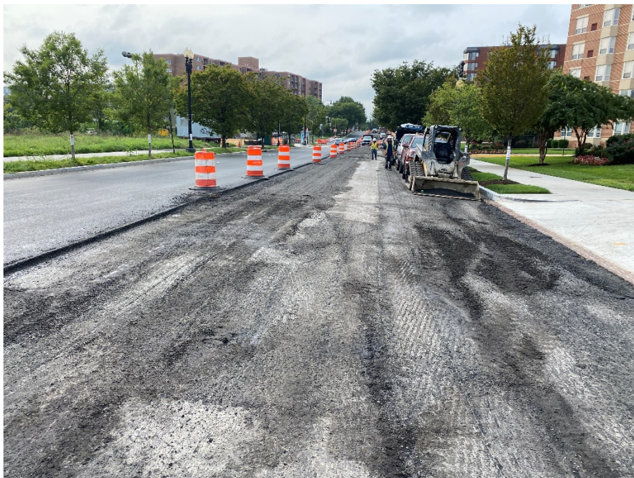
Picture No. 12 – 09/18/2020 – Pavement milling along NJ Ave between K St. and NY Ave. (South View)
