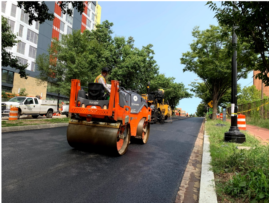
Picture No. 5 – 09/15/2020 – Placement of HMA along NJ Ave between H St. and I St. (North View)
