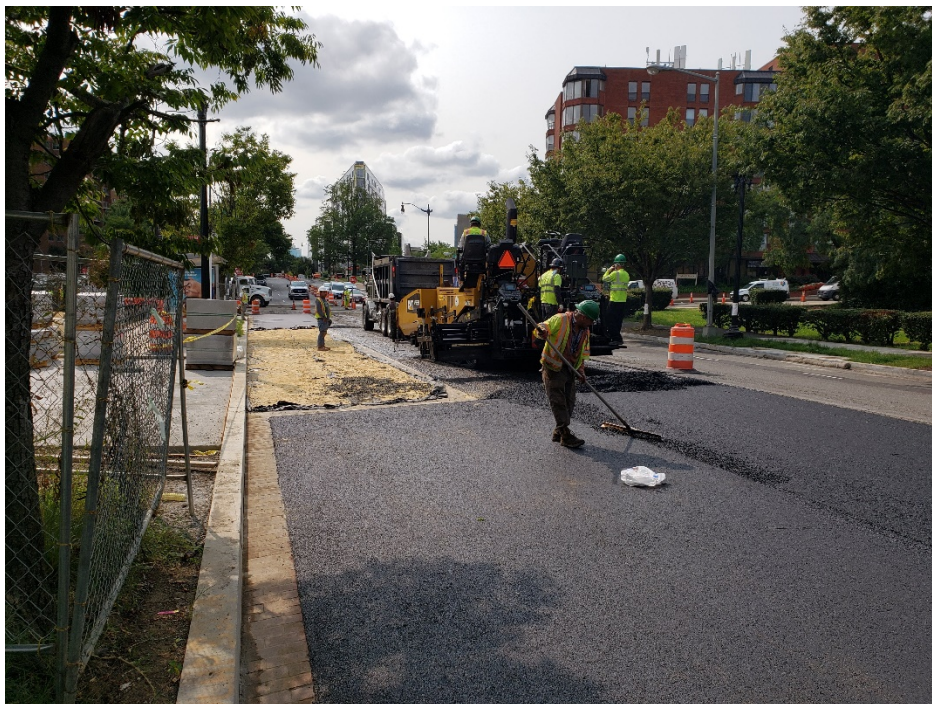
Picture No. 8 – 09/16/2020 – Placement of HMA along NJ Ave between K St. and NY Ave (South view)
