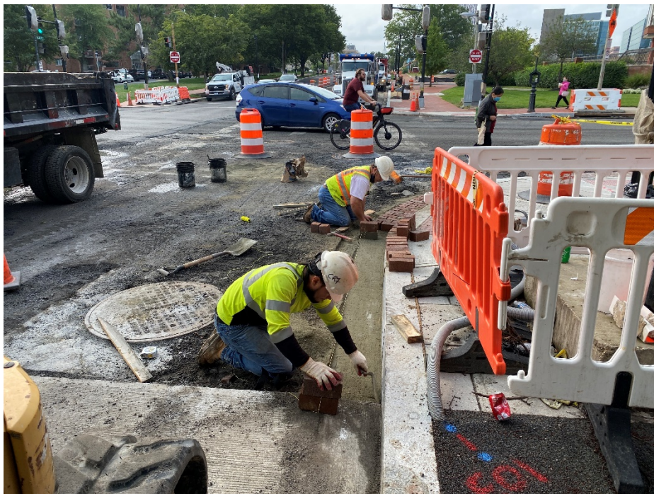
Picture No. 14 – 09/18/2020 – Repairs to brick gutter along NJ Ave at K St. and NY Ave. (North View)
