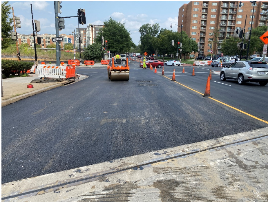
Picture No. 13 – 09/18/2020 – Placement of HMA at the intersection of NJ Ave and K St. (North view)
