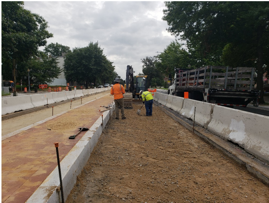
Picture No. 11 – 09/17/2020 – Grading of aggregate base course along NY Ave between 1 st St. and NJ Ave (West view)
