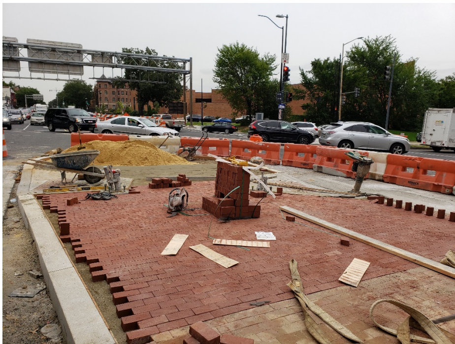
Picture No. 10 – 09/17/2020 – Installation of brick median in progress at NY Ave and 4 th St. intersection (East View)
