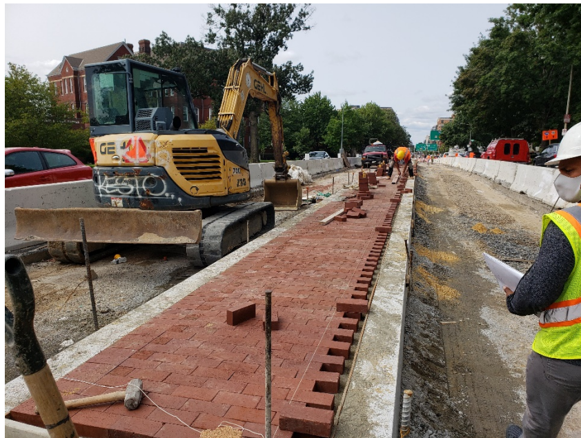
Picture No. 2: 09/14/2020 – Placement of brick median along NY Ave between 1 st St. and NJ Ave. (West View)
