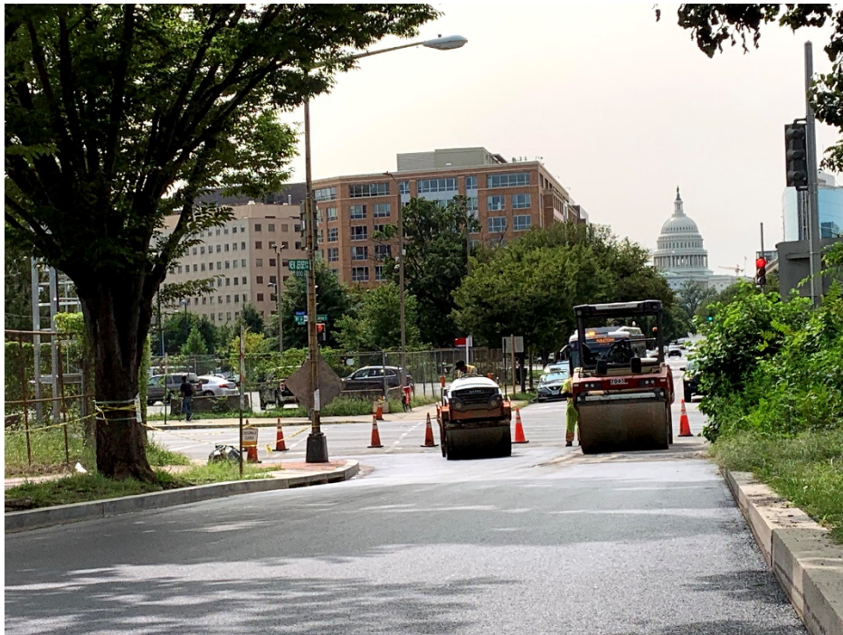
Picture No. 6 – 09/15/2020 – Placement of HMA along NJ Ave between H St. and I St. (South View)
