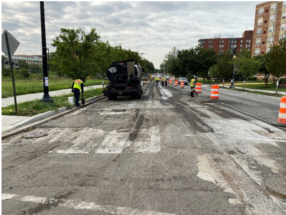
Picture No. 7 – 09/16/2020 – Installation of tack coat along NJ Ave between K St. and NY Ave. (South View)
