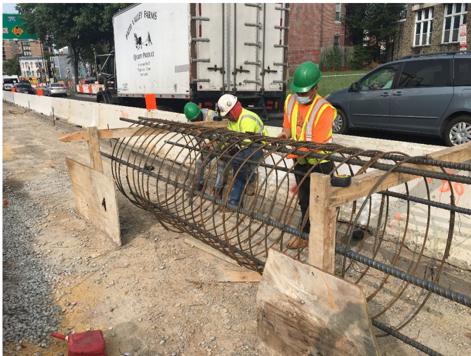
Picture No. 4 – 09/15/2020 – Drilled shaft rebar cage for the overhead sign structure along NY Ave and Kirby St. (East View)
