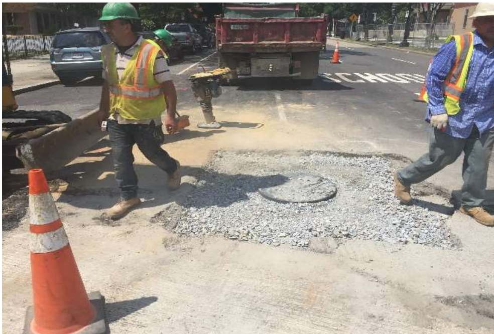
08/01/2019 – Installing Manhole #8 at NJ Ave.NW across from the Library.
