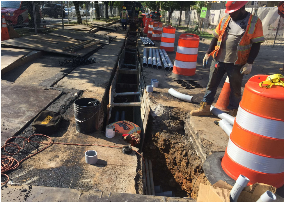
08/01/2019 – Installing conduits for electric duct bank at NJ and I St. NW
