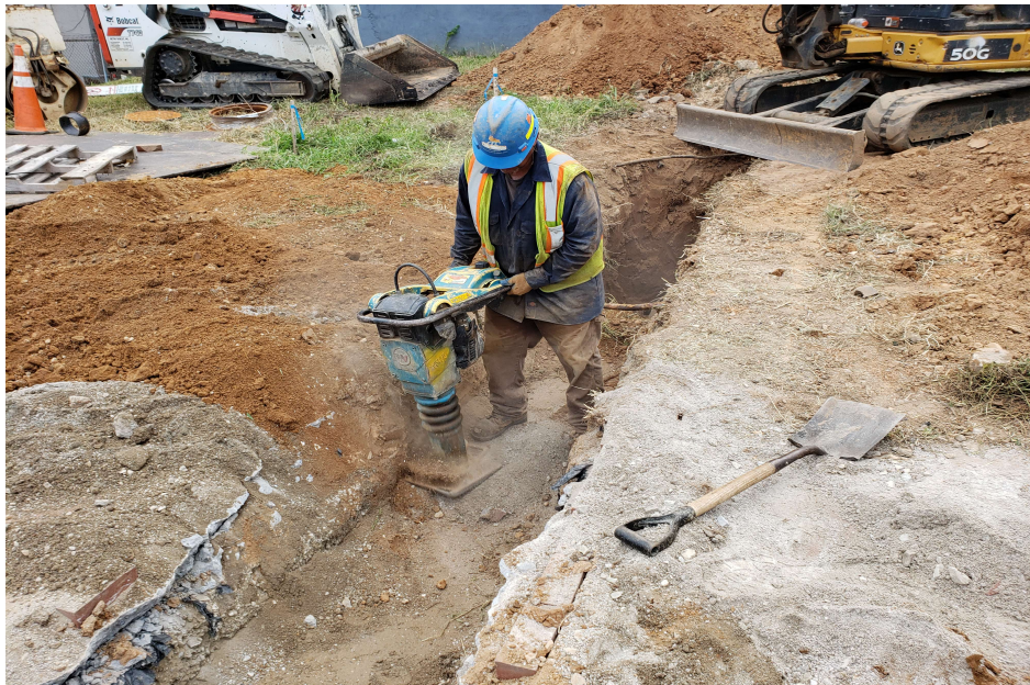
07/29/2019- Compaction to the soil backfill for 8" DIP water main at 3 rd & M St. NW. (SW Corner)
