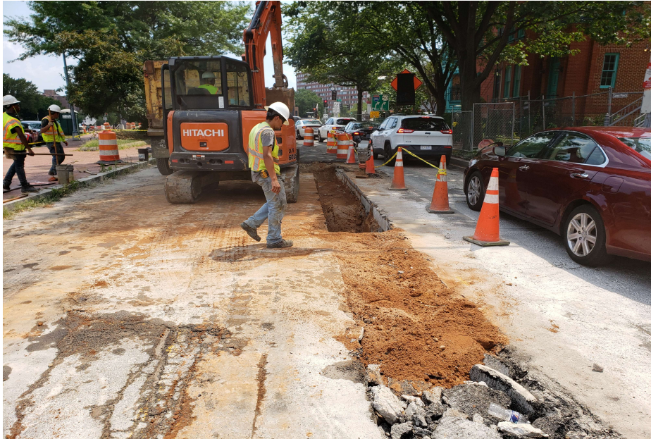
07/29/2019 – Installing 8" DIP water main at 3 rd St. NW near M St. NW.
