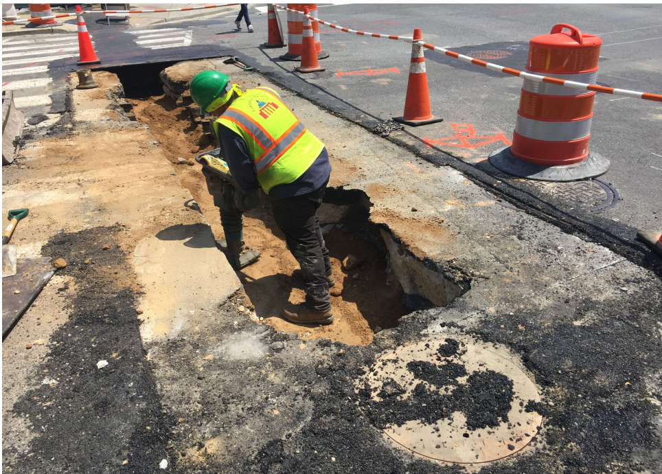
07/30/2019 – Compaction to the trench line at NJ Ave. and K St. NW.
