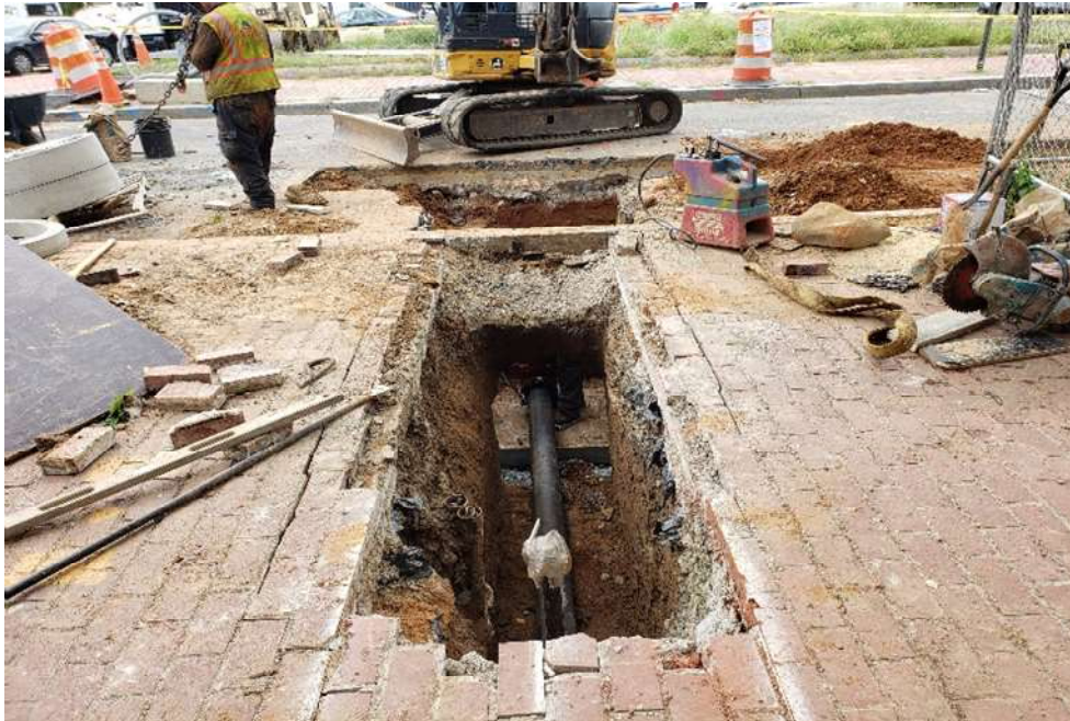
07/31/2019 – Installing 8" Water main at intersection of NJ. And NY Ave. NW
