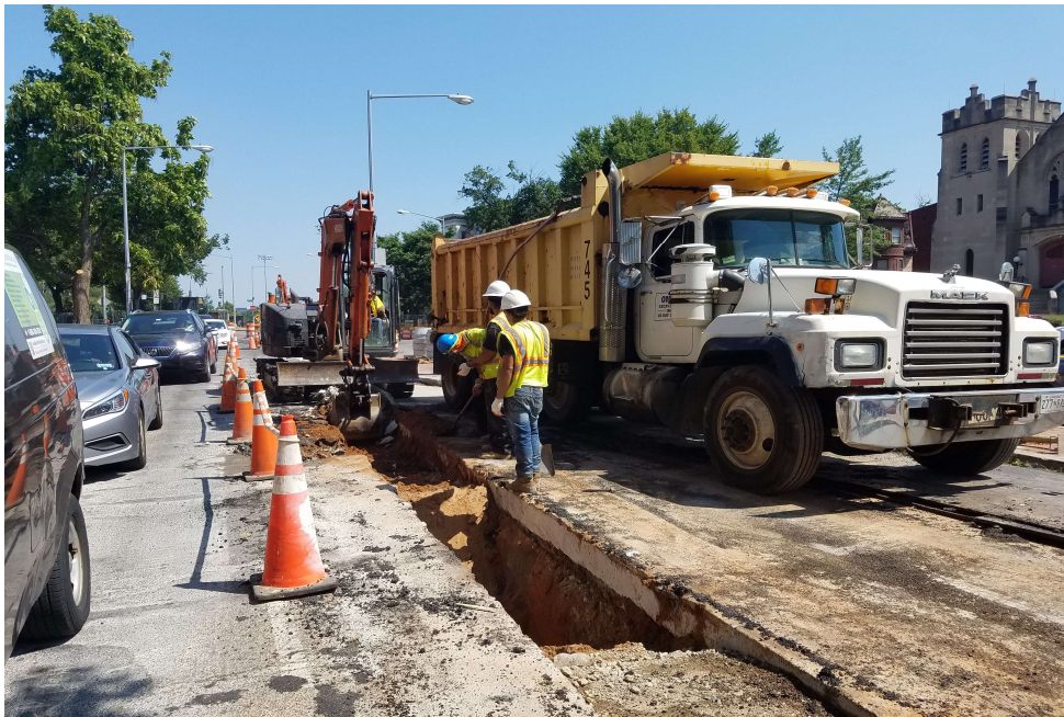
07/30/2019- Installing 8" DIP water main at intersection of M and 3 rd St. NW.
