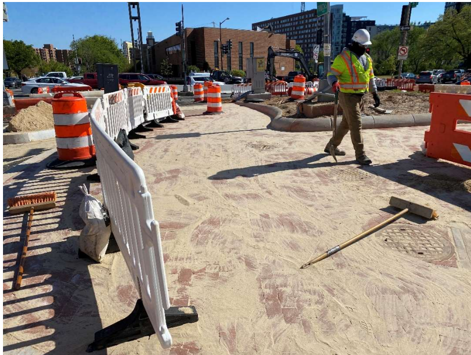
Picture No. 7 - 04/22/2020 - Sweeping fine sand into joints of brick sidewalk near the intersection of NJ Ave and M St (South View)
