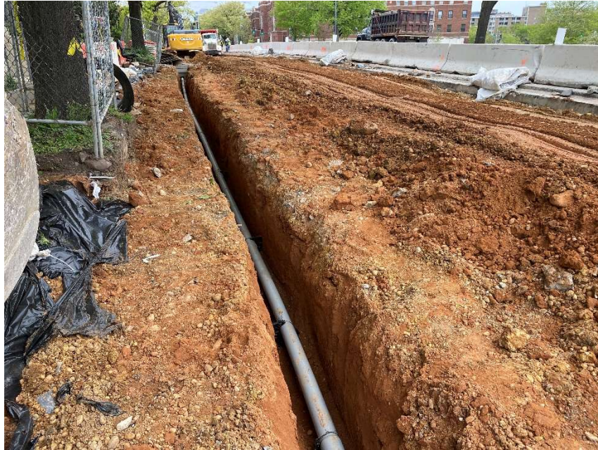
Picture No. 1: 04/20/2020 – Installation of electrical duct bank for OHV detection system in progress along NY Ave between 1 st St. and Kirby St. (East View)
