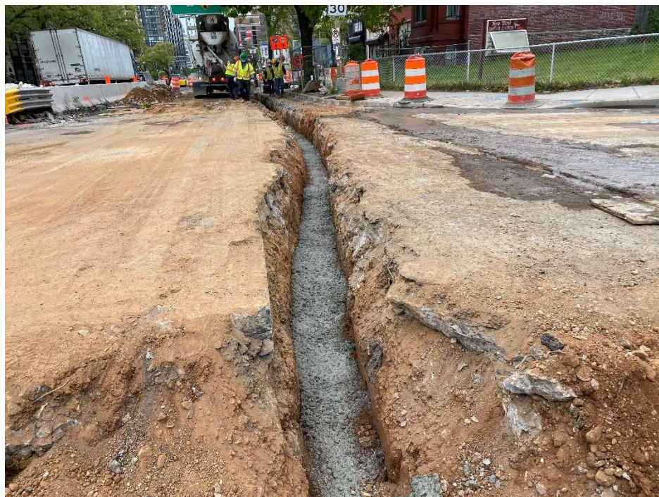
Picture No. 8 – 04/23/2020 – Encasement for electrical duct bank for OHV detection system at NY Ave Kirby St. (West View)
