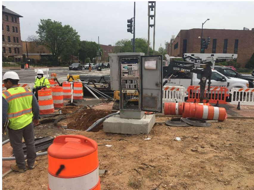
Picture No. 2: 04/20/2020 – Relocation of traffic cabinet onto temporary base at the NJ Ave and NJ Ave intersection (South View)
