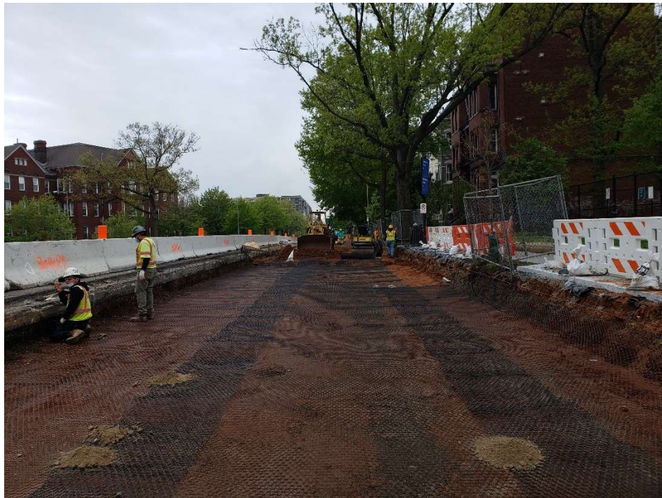
Picture No. 3 - 04/21/2020 – Geogrid placement on westbound NY Ave between First St and Kirby St (West View)
