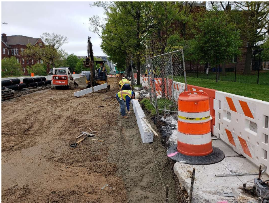
Picture No. 10 – 04/25/2020 – Furnish and setting granite curb along NY Ave between 1 st St. and Kirby St. (West View)
