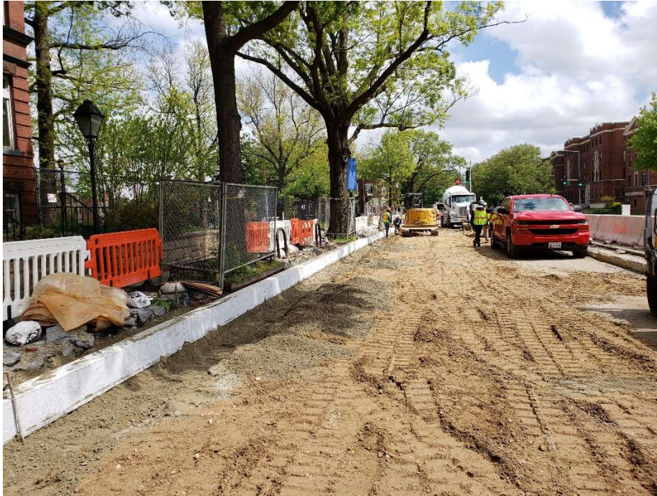
Picture No. 11 - 04/25/2020 – Furnish and setting granite curb along NY Ave between Kirby St. and NJ Ave (East View)
