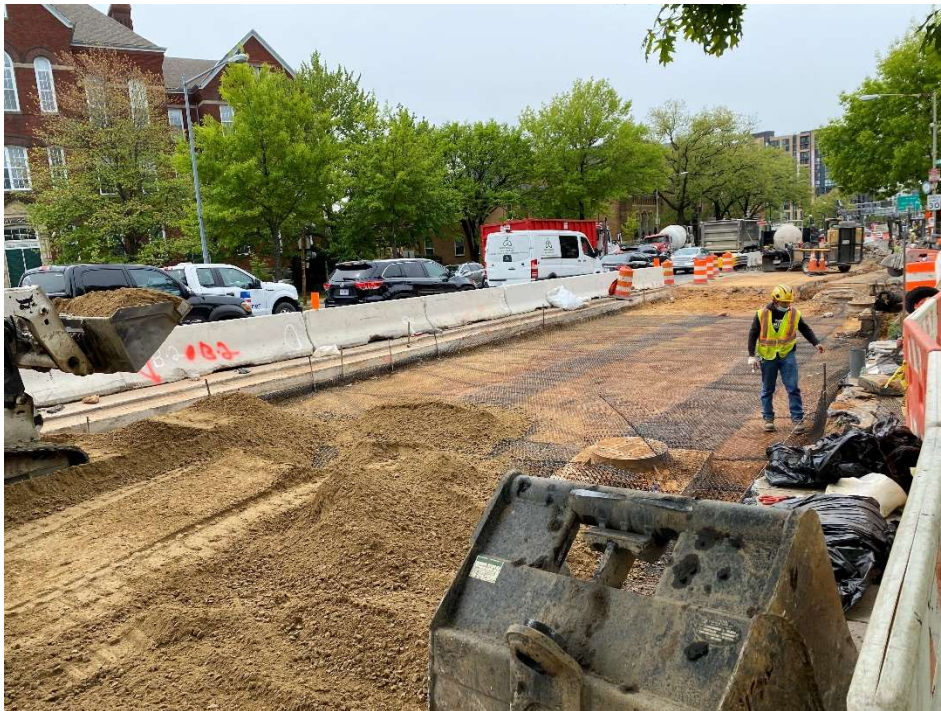
Picture No. 9 - 04/23/2020 – Ongoing placement of geogrid and aggregate base course NY Ave between Kirby St. and NJ Ave (West View)
