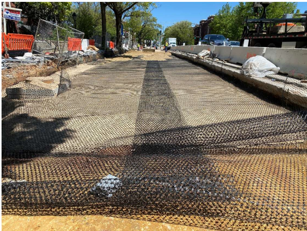
04/22/2020 – Geogrid placement westbound NY Ave between 1 st St. and Kirby St. (East View)
