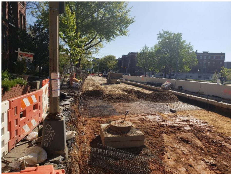
Picture No. 6 – 04/22/2020 – Installation of geogrid and aggregate base on NY Ave between 1 st St. and Kirby St. (West View)
