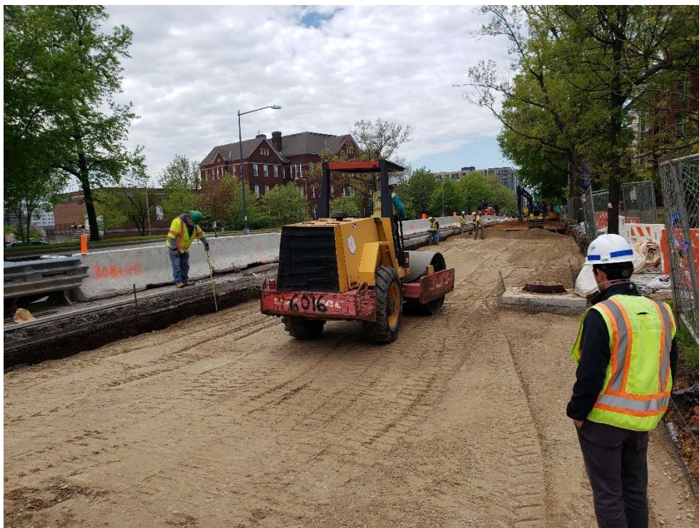
Picture No. 4 – 04/21/2020 – Placement and installation of aggregate base course near NY Ave and 1 st St. (West View)
