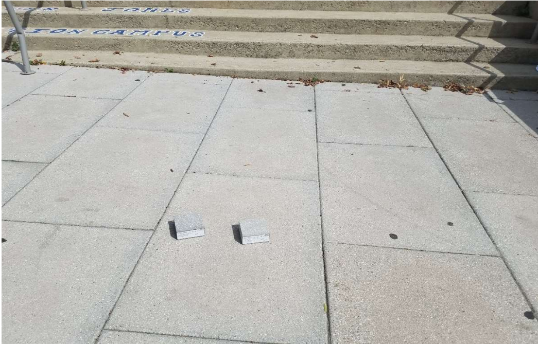
09/17/2019- Samples of Block sidewalk to check similarity with the existing one at East Side of NJ Ave NW, North of L St. (East View)
