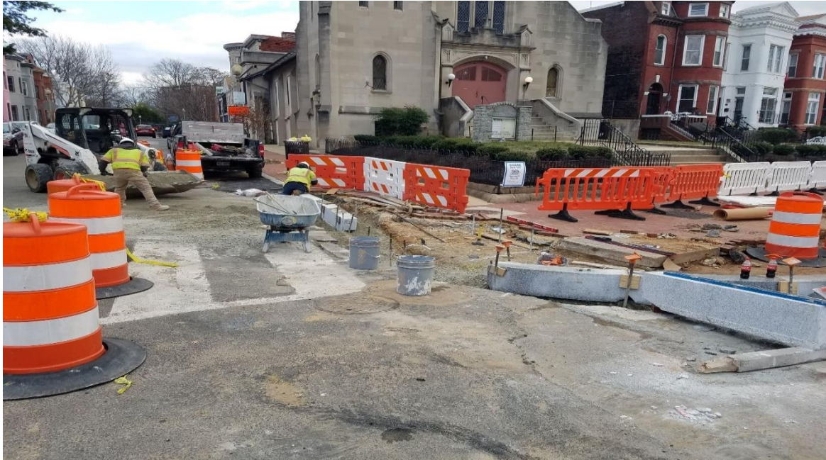
01/27/2020- Furnish and set granite straight curb at South side Morgan St & NJ Ave NW. (E. view)
