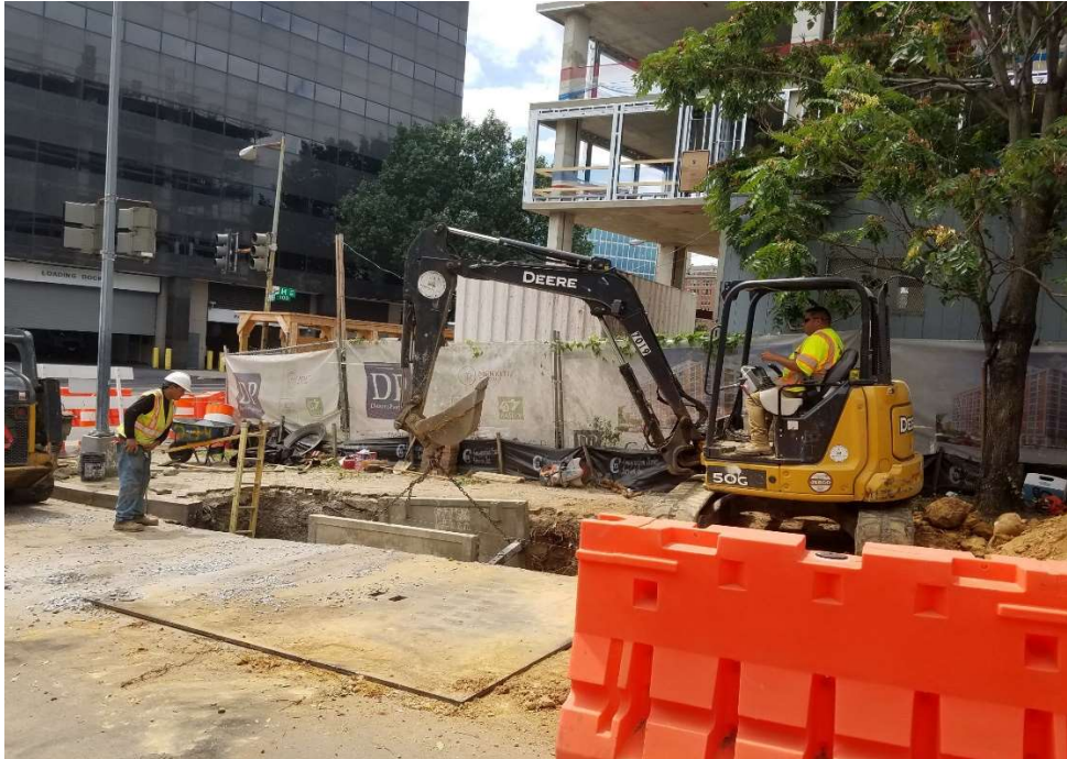
08/14/2019 – Safety measures to the trench excavated for catch basin installation at NW corner of NJ & H St. NW(West View)
