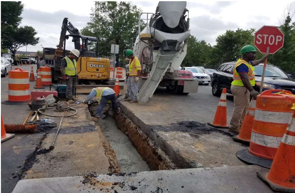
08/15/2019 – Concrete pouring on Street light conduits at NJ & 2 nd St. NW. (South View)
