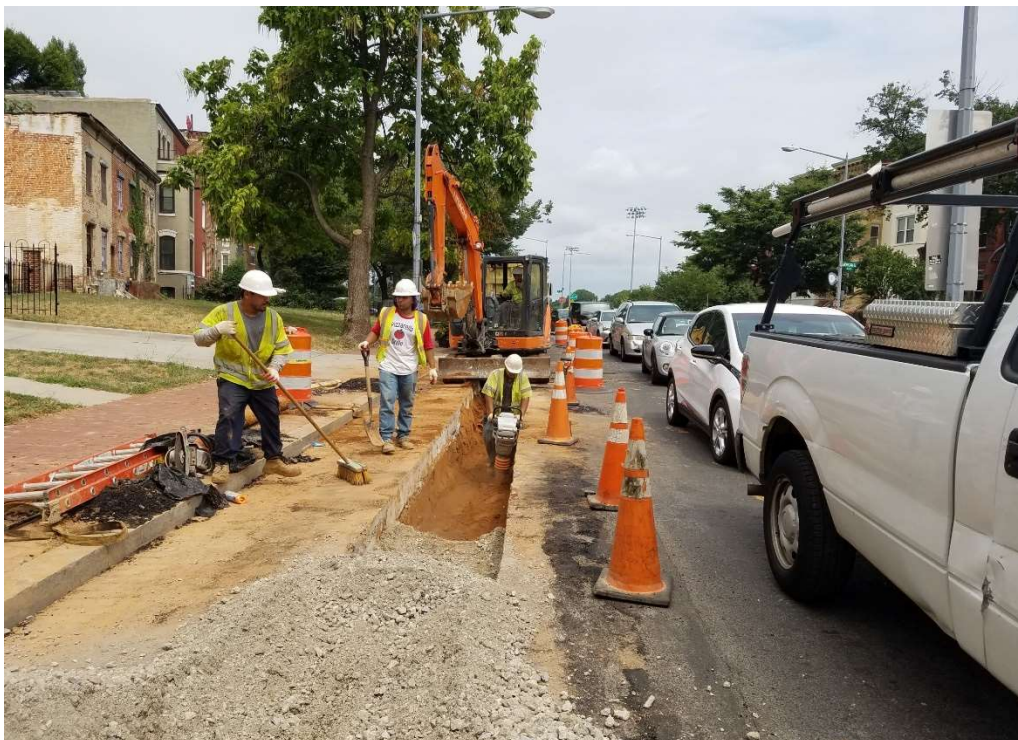
08/15/2019 – Backfill/compaction to 8" DIP water main at 3 rd St. NW btwn NJ & M St. NW. (North view)
