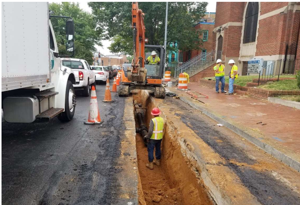
08/13/2019 – Installing 8" DIP water main line along 3 rd St. NW between M & NJ Ave. NW. (South View)
