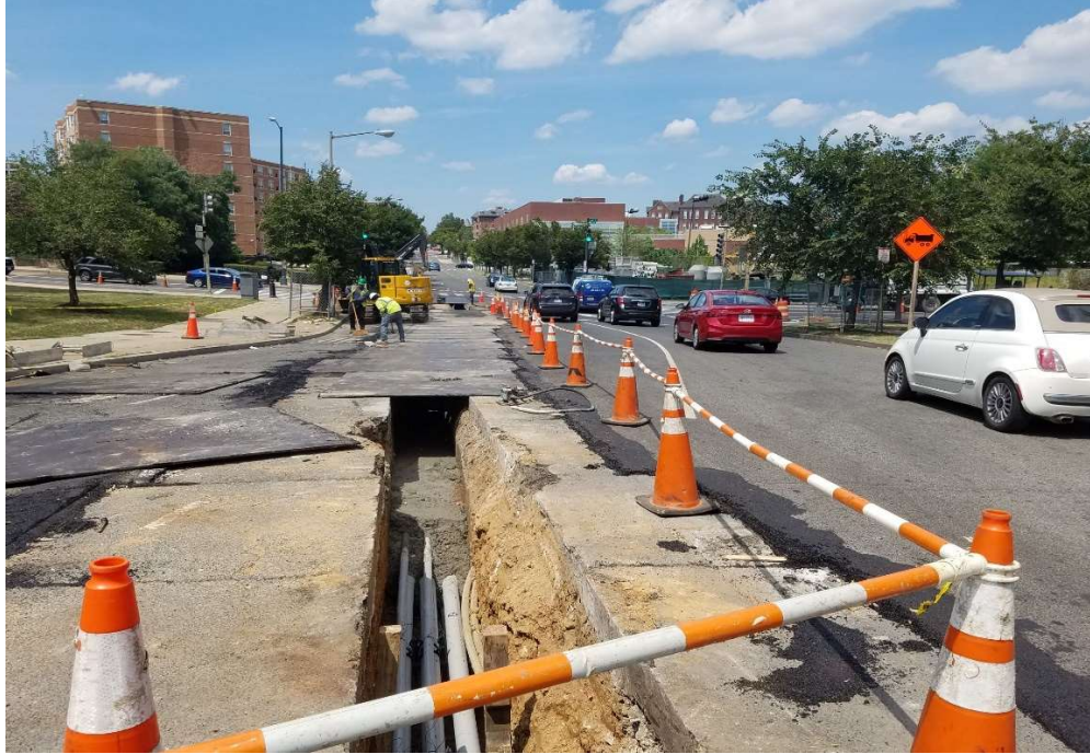
08/12/2019 – PVC conduits installed at West side NJ Ave. NW between K & I St NW (North View)
