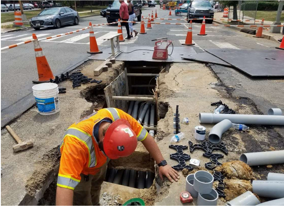
08/15/2019- Installing electric conduit at/near NJ & K St. NW (South View)
