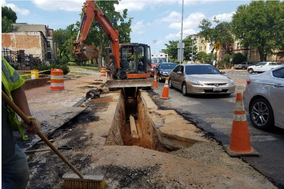
08/12/2019 – Installing 8" DIP water main at 3 rd St. NW between M St. & NJ Ave. NW (North View)
