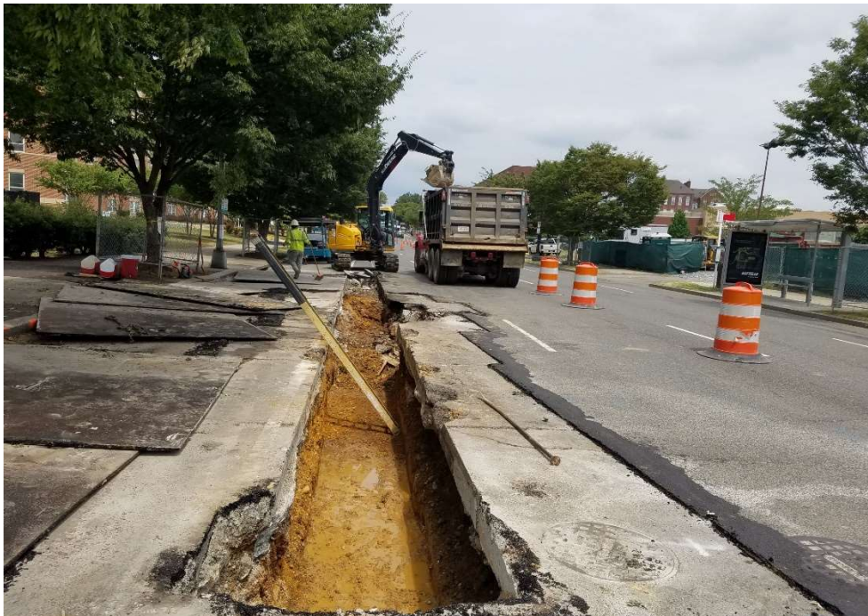
08/15/2019-Trench excavation for traffic signal at West side of NJ Ave. between K & L St. (North View)
