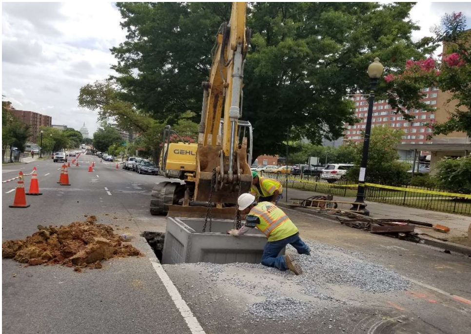
08/14/2019 – Installing 4'x4'x4' Streetlight MH at West side of NJ Ave near Pierce St. NW (South View)
