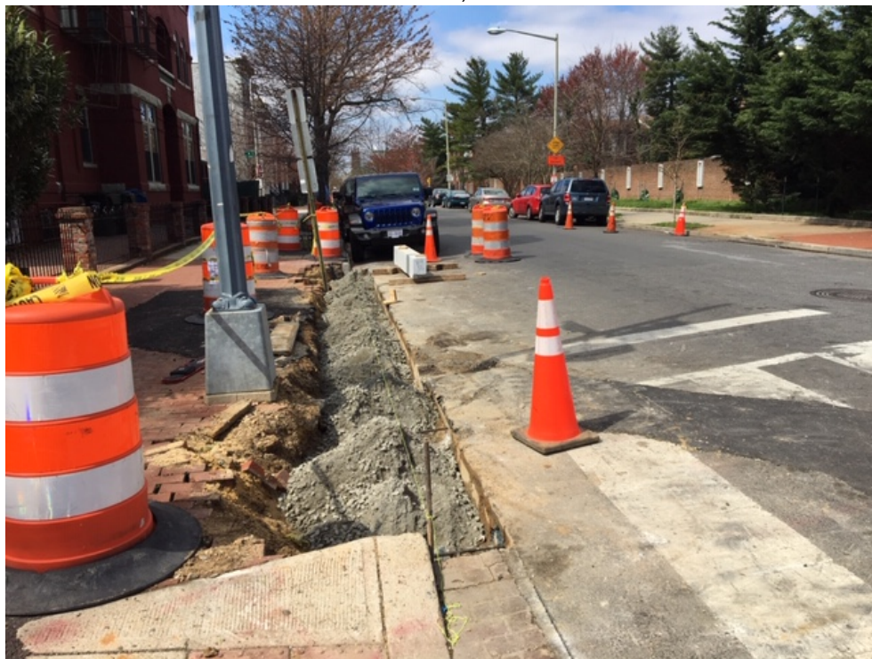
Picture No. 4 - 03/26/2020 – Placement of dry mix for installation of the granite curb along N St. (West View)
