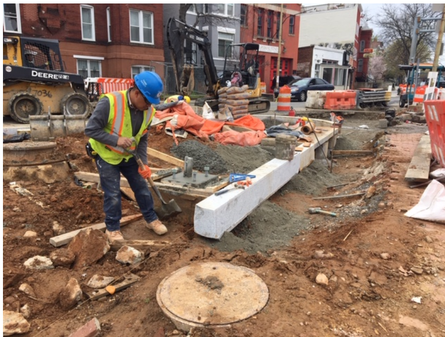
Picture No. 1: 03/24/2020 - Installation of the granite curb along M St. east of NJ Ave and M St. intersection adjacent to the island (East View)
