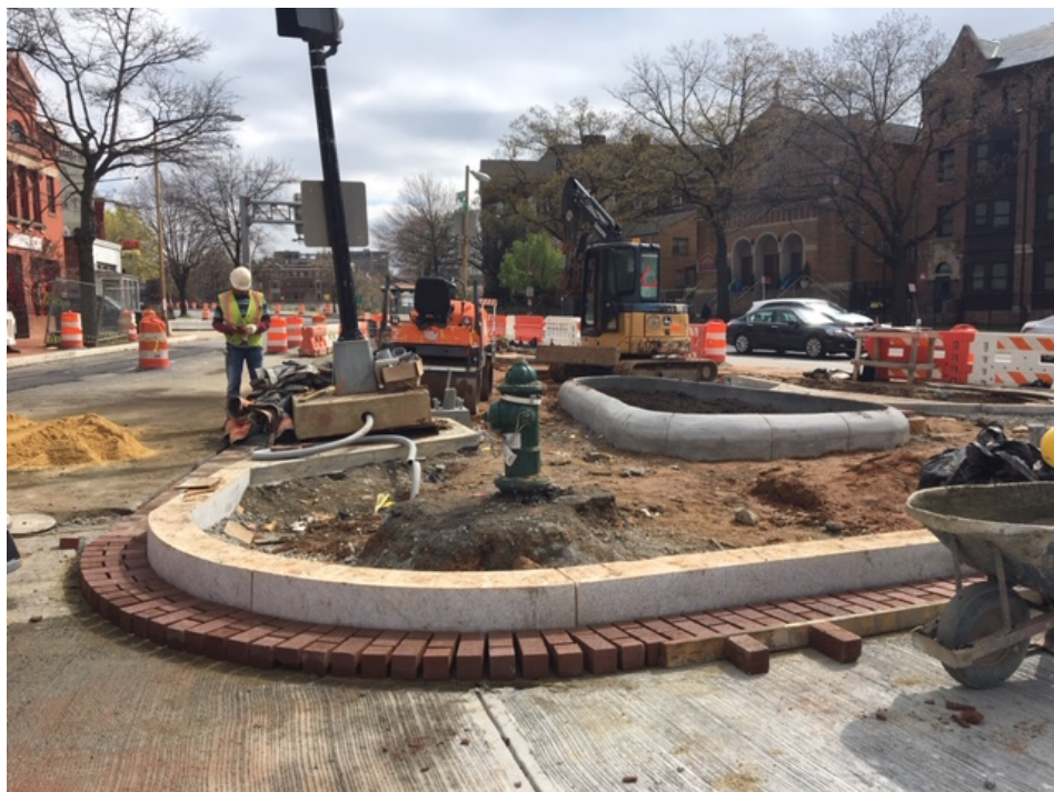
Picture No. 6 - 03/26/2020 – Installation of the brick gutter along M St. east of NJ Ave and M St. intersection adjacent to the island (East view)
