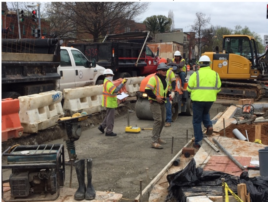
Picture No. 2 - 03/24/2020 – Placing and compacting aggregate base for PCC base placement at the NE corner of NJ Ave and M St (North View)
