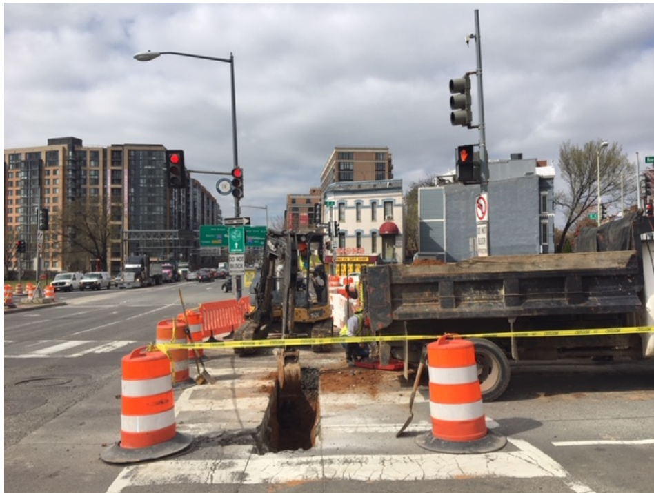
Picture No. 5 - 03/26/2020 – Trench excavation for conduit duct bank at the intersection of NY Ave and NJ Ave (West View)
