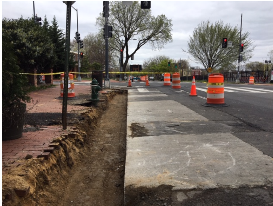
Picture No. 3 - 03/24/2020 – Excavation in progress for granite curb installation along NJ Ave and N St. (North View)
