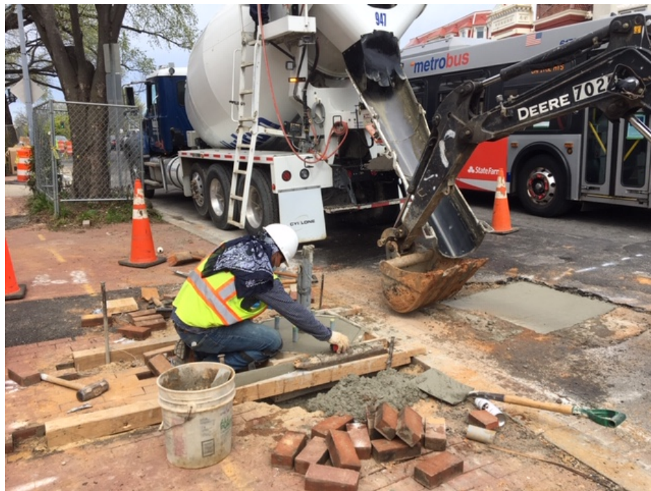
Picture No. 8 - 03/27/2020 – Installation of PCC streetlight foundation at the intersection of NJ Ave and Morgan St. on SB travel lane (South View)
