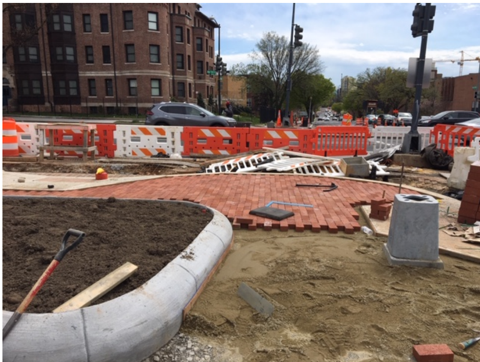
03/27/2020 – Installation of the brick side at the intersection of NJ Ave and NY Ave NE island (South View)
