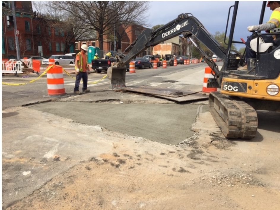
Picture No. 7 - 03/27/2020 – Installation of PCC base at the intersection of M St and NJ Ave. (North View)
