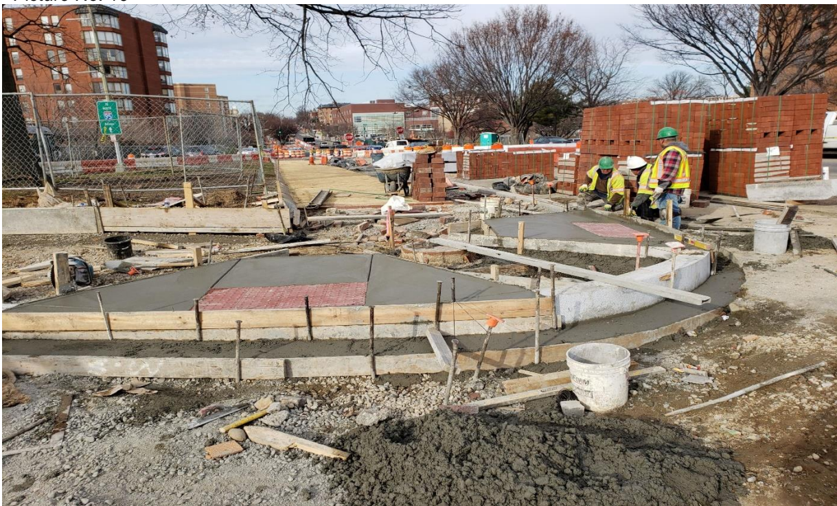
01/10/2020 – Wheelchair ramp constructed at NW corner of NJ Ave. and I St. NW.
