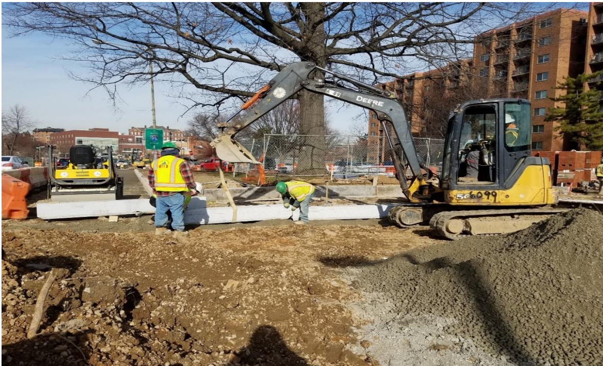
01/09/2020- Installing Granite Straight Curb at 2 nd & I St. NW North side. ( North View)
