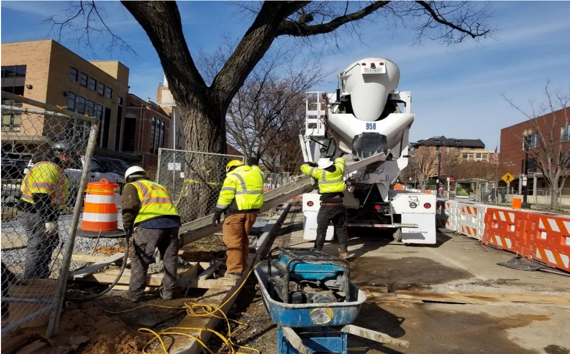
01/09/2020 - Concrete pouring for Pole foundation at West side of NJ Ave. NW in front of Bible church. (North view)
