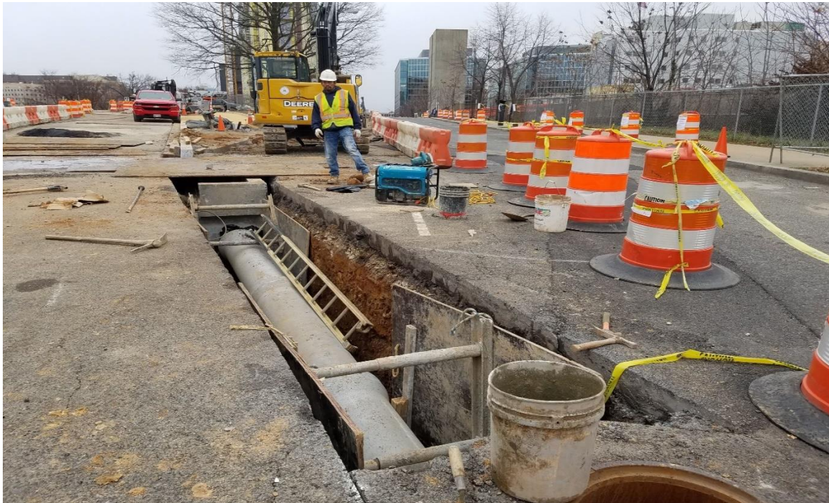
01/07/2020- 18" RC Pipe installed to connect Catch Basin U1A and Manhole U2 (South view)
