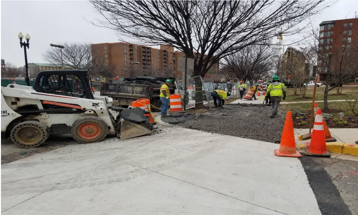
01/07/2019- Removal of deficient flexi-pave area at West side of NJ Ave. NW, North of K St. (S. View) Picture No. 6
