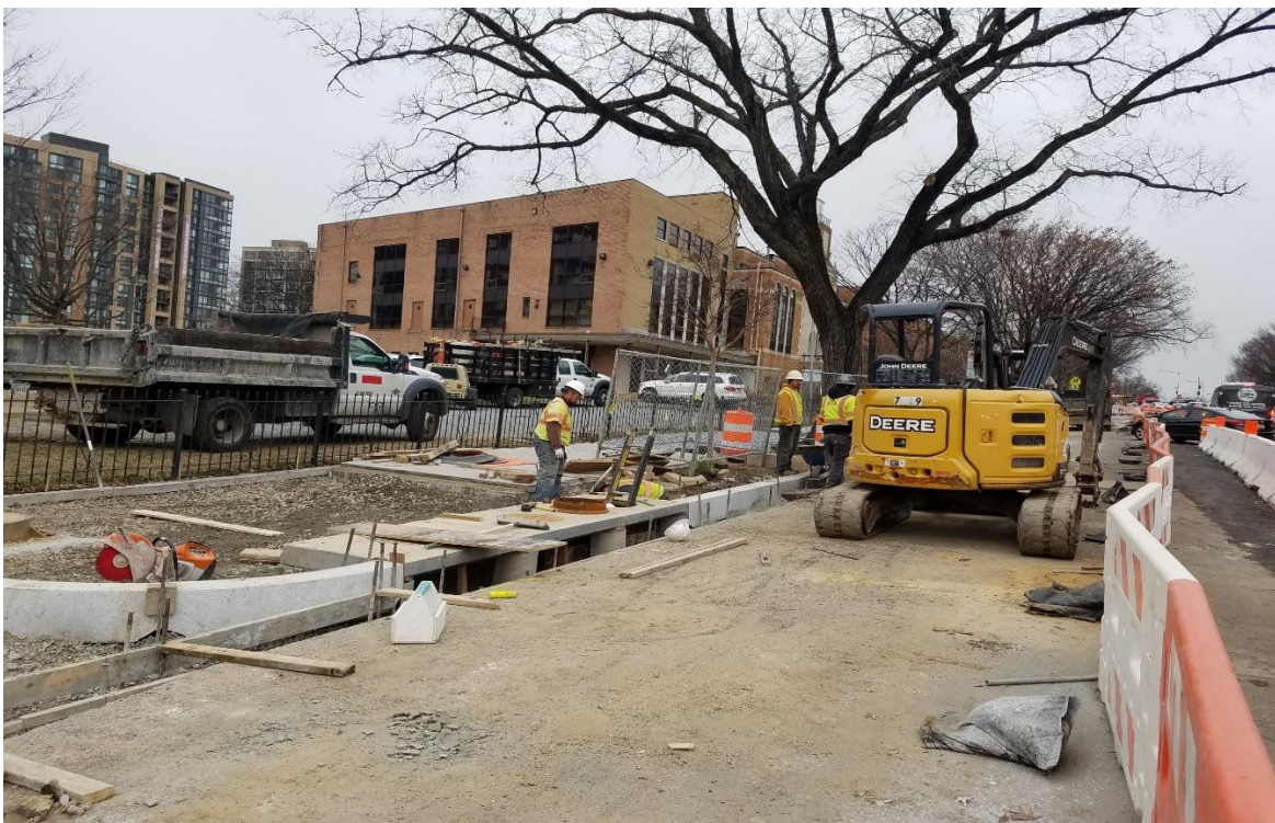
01/07/2020- Triple catch basin (Structure O) installed at East side of NJ Ave. NW b/n L & Pierce St.
