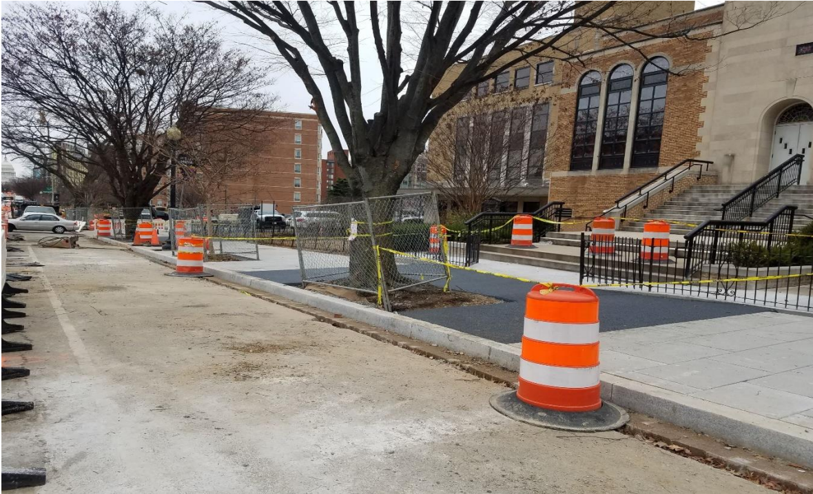
01/07/2020- Flexi pave sidewalk constructed at NJ Ave. NW in front of Bible Way Church. (SW view)
