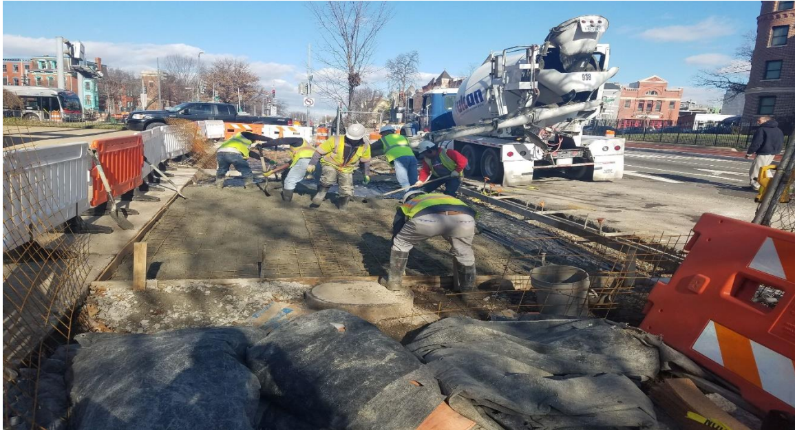
01/06/2020- Repair/replace driveway at North entrance of Bible Way Church at NJ Ave b/n L & NY Ave NW. (North View)
