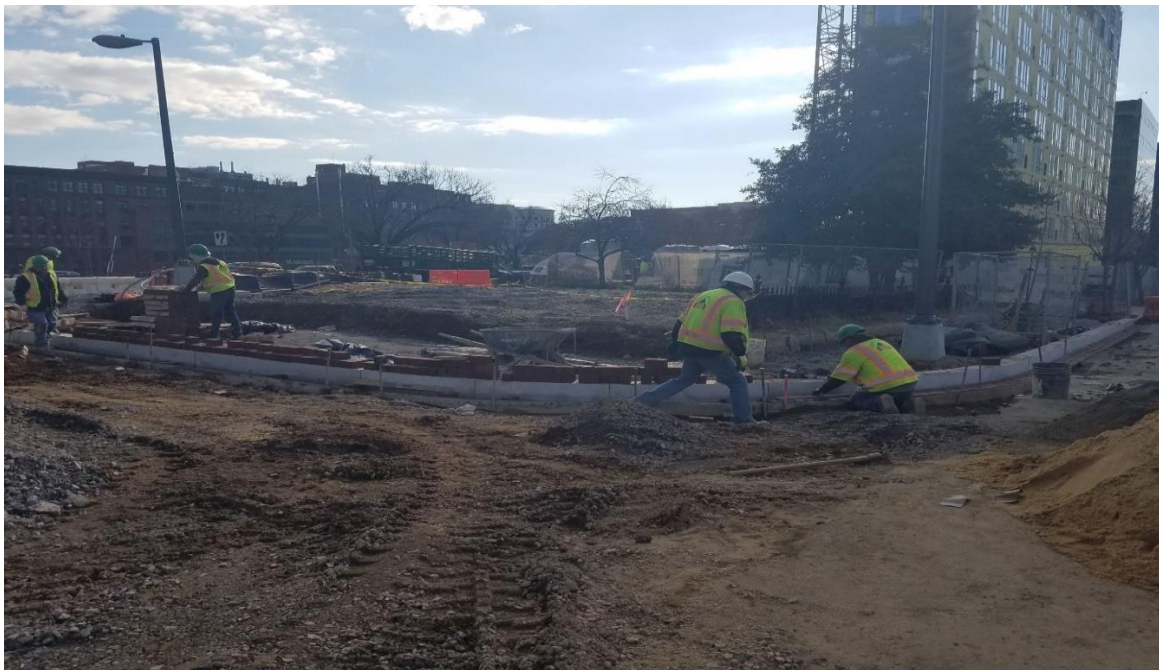
01/06/2020 – Brick gutter construction at 2 nd & I St. NW. (South view)
