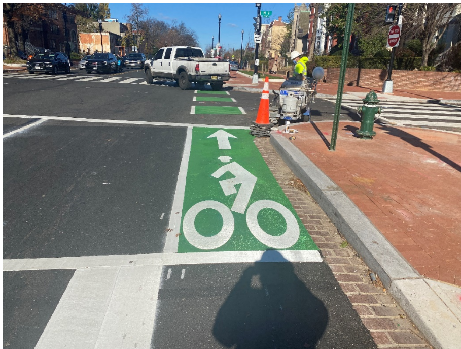
Picture No. 2: 11/23/2020 – Installation of pavement marking along NJ Ave between M St. and N St. (North View)
