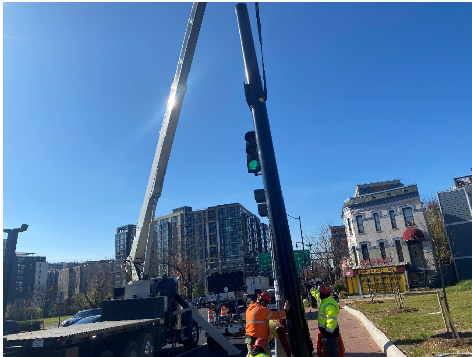
Picture No. 5 – 11/24/2020 – Installation of vertical element of the monotube pole along NY Ave and NJ Ave intersection – NW corner (West View)
