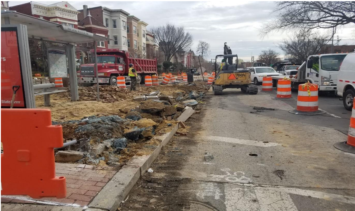
02/04/2020 – Removal of existing curb & island at/near New Jersey Ave. & 3 rd St. Intersection. (South View) Picture No. 4
