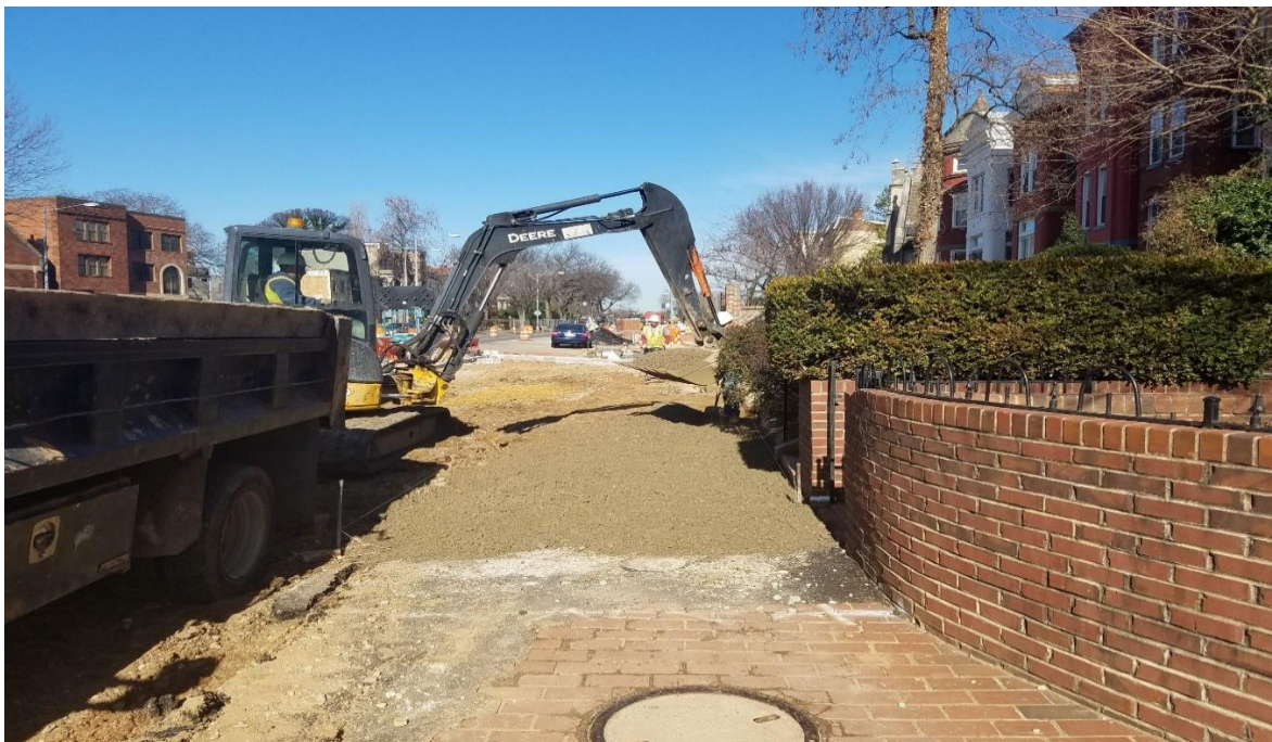
02/03/2020- GAB placement for sidewalk at East side of NJ Ave. NW b/n NY Ave. and Morgan St. NW. (N. view)
