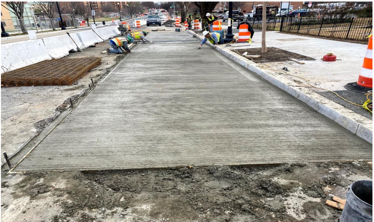
02/08/2020- Finishing work on PCC bus pad constructed at West side of NJ Ave. NW Near Pierce St. (South View)
