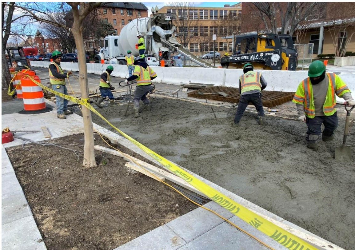
02/08/2020 - PCC Bus pad construction at West side of NJ Ave. NW Near Pierce St. NW. (NE view.)
