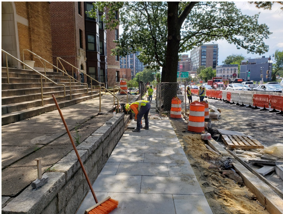
Picture No. 4 – 07/28/2020 – Installation of block paver on PCC base along NY Ave between NJ Ave and M St. (West View)
