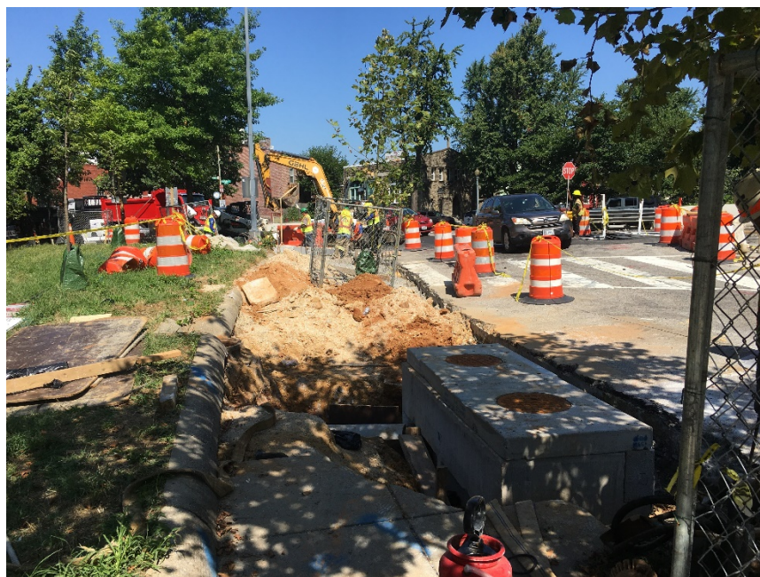
Picture No. 1: 07/27/2020 – Installation of Catch Basin and excavation around the basin along M St. and NY Ave. (West View)
