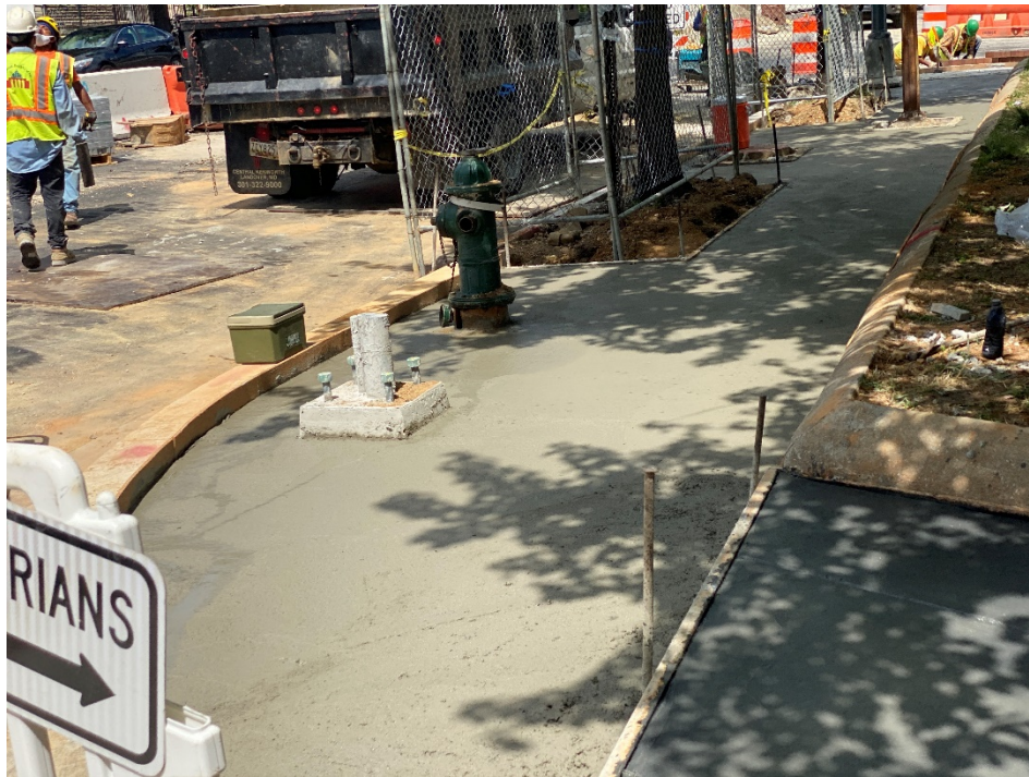
Picture No. 3 - 07/28/2020 – PCC installation for block pavers along NY Ave and M St. intersection (East View)
