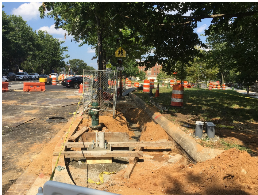
Picture No. 2: 07/27/2020 – PCC base installation for the pole foundation along NY Ave and M St. intersection (East View)
