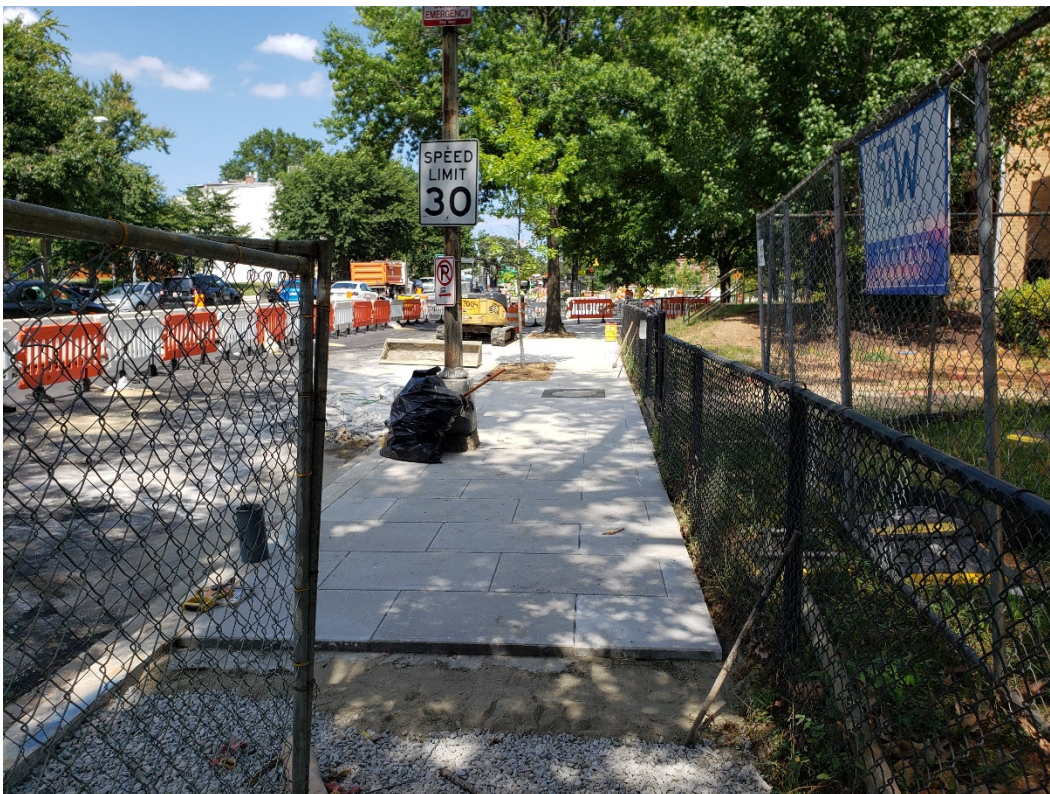
07/28/2020 – Installation of block pavers sidewalk along eastbound NY Ave between Kirby St. and M St. (East View)
