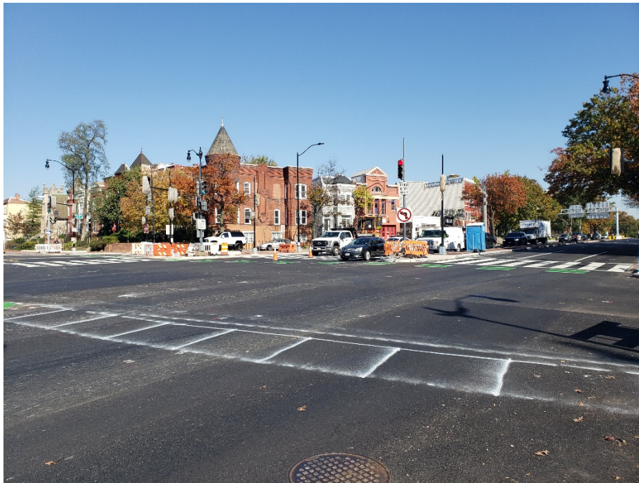
Picture No. 9 – 11/06/2020 – Pavement marking layout in progress at the intersection of NY Ave and NJ Ave (West view)
