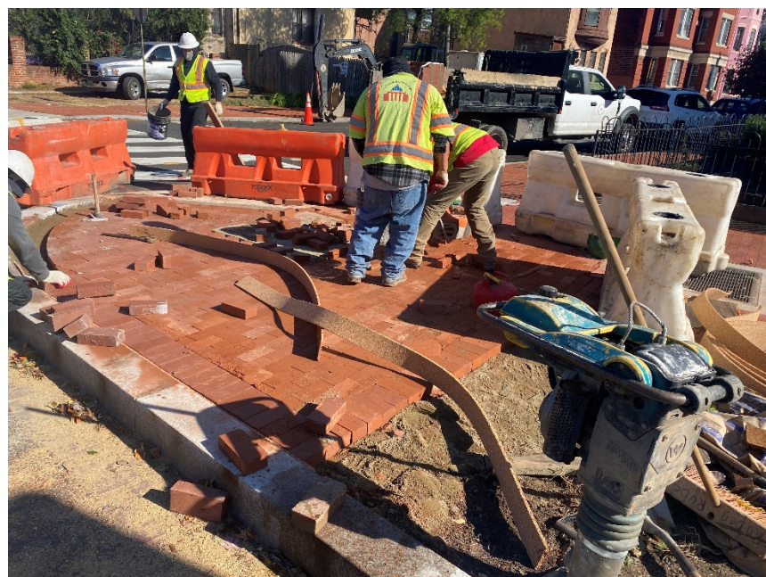
Picture No. 2: 11/02/2020 – Brick sidewalk installation in progress along NJ Ave and Morgan St. (Northeast View)
