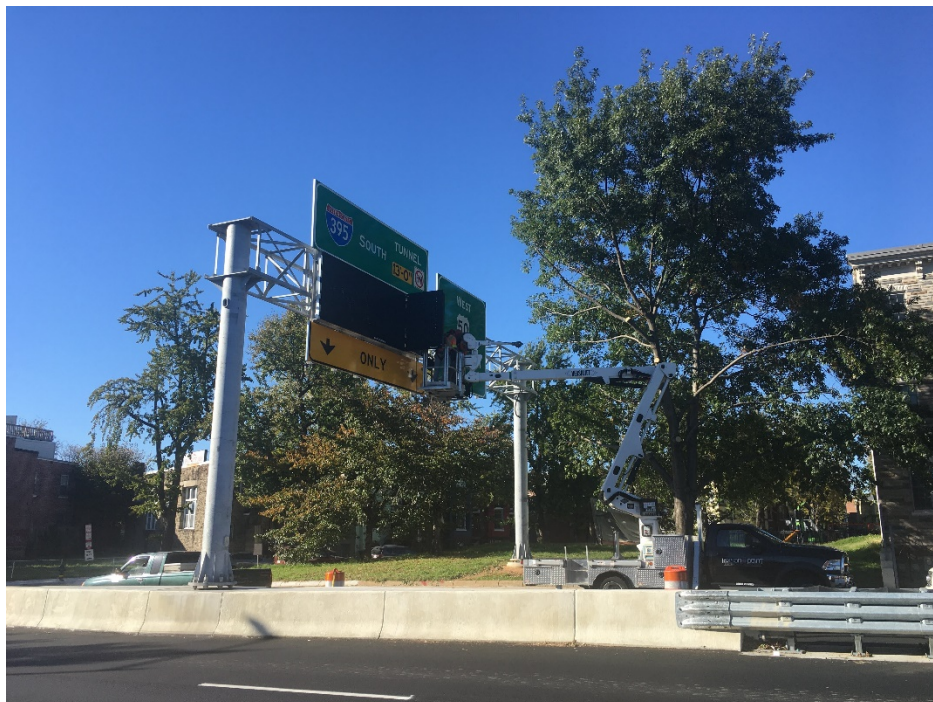
Picture No. 6 – 11/04/2020 – Jaxon Point crew working on the DMS board along NY Ave and Kirby St. (North View)
