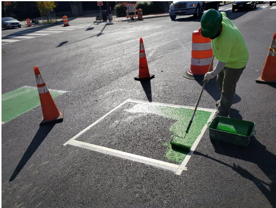
Picture No. 7 – 11/05/2020 – Pavement marking in progress along NY Ave and NJ Ave intersection (East View)
